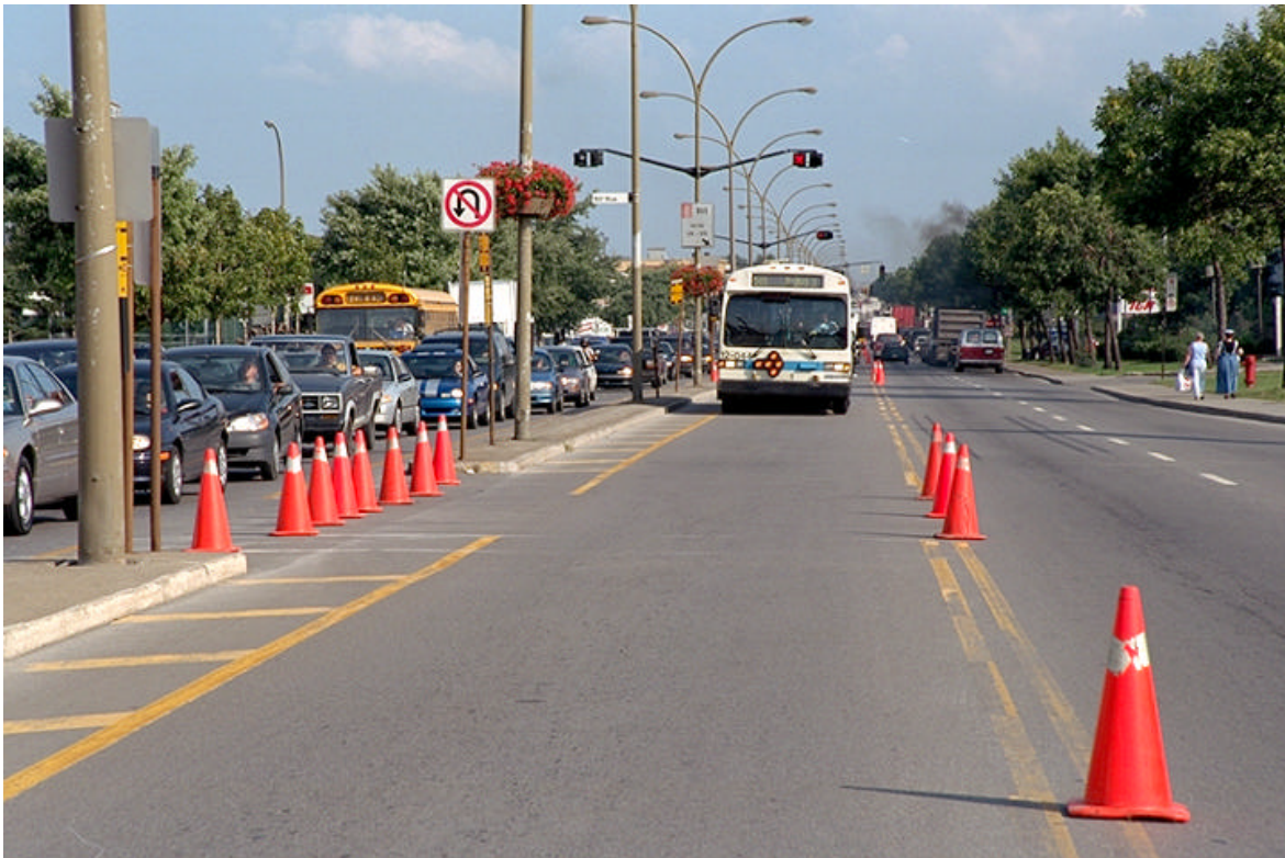
Pie IX Boulevard Contraflow Bus Lane - Montreal
