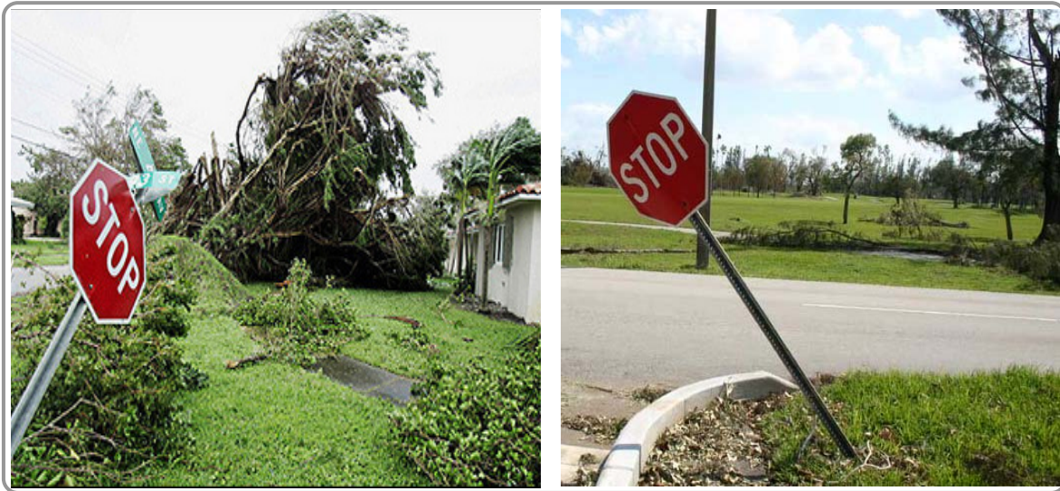
Figure A: Stop signs damaged in Miami-Dade County during Hurricane Wilma
