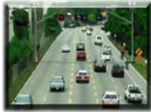
This reversible lane project on Sepulveda Boulevard in Los Angeles uses overhead signals to control traffic in the specially marked lane
