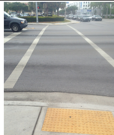
Pavement markings are fair and ADA pedestrian ramps exist at all corners.
