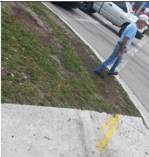
SE corner of W 28 Ave and W 68 St: Tire marks cutting into return and pedestrian ramp
