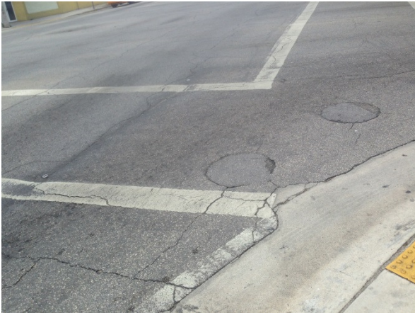
Cracked and faded paving markings.
