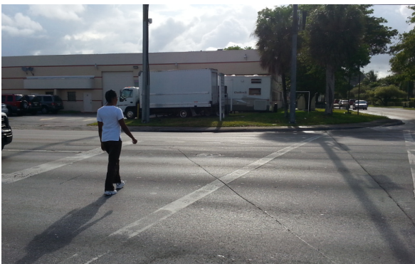
W 28 Ave North Leg: Un-signalized pedestrian crossing/faded markings.
