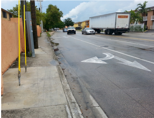
W 24 Ave Northbound: Drainage issue; sand is visible all the way up to the NW return of the intersection.
