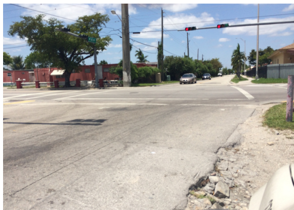
Southeast corner: angle parking damages the edge of pavement.
