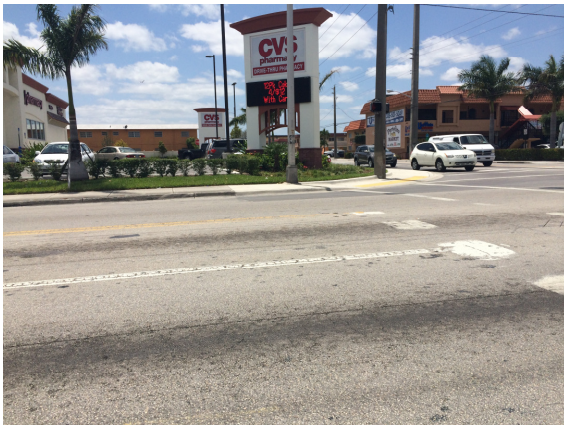
Faded pavement markings.
