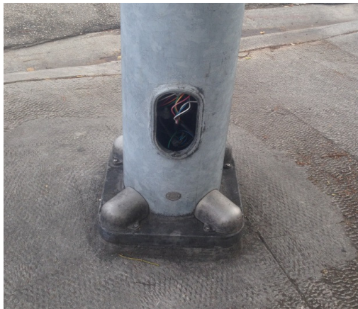
South-East corner: Mast arm post in substandard conditions.
