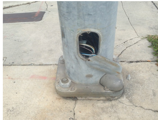
North-East corner: Mast arm post in substandard conditions.
