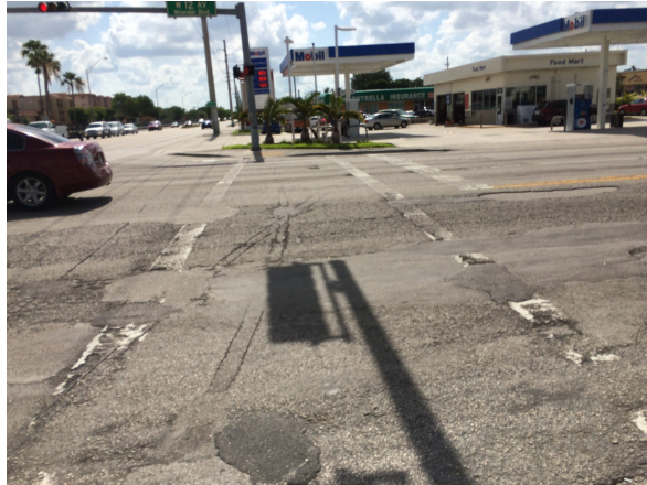
Deteriorated pavement conditions.
