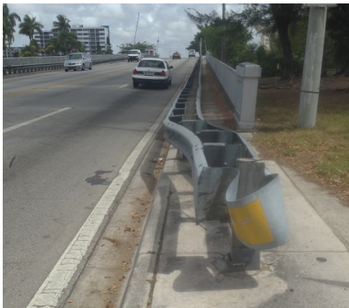
Damaged guardrail
