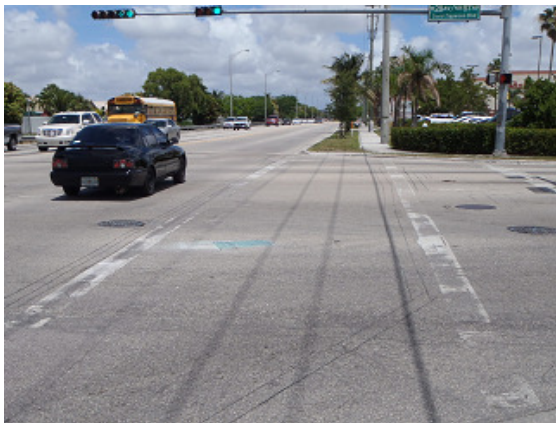
W 68 St Eastbound: Faded Pavement markings.
