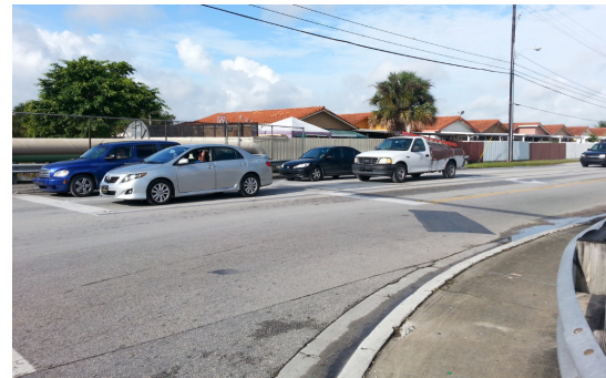
W 76 St west leg: Staggered stop bar.
