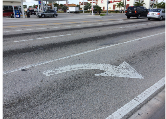
Faded pavement markings and deteriorated pavement conditions.
