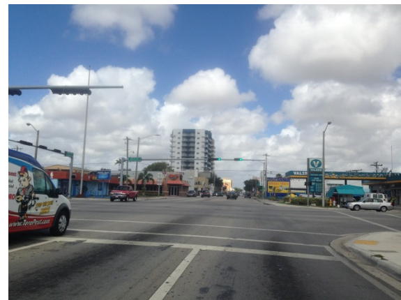
Westbound approach: Signals heads poorly visible.
