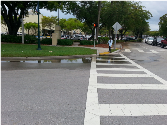
Water ponding on SE corner in front of ramp.
