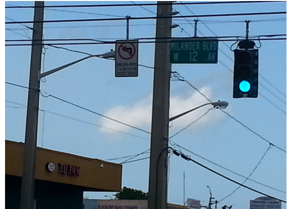
Span wire signal, and turn restrictions during peak hours for east/west traffic.
