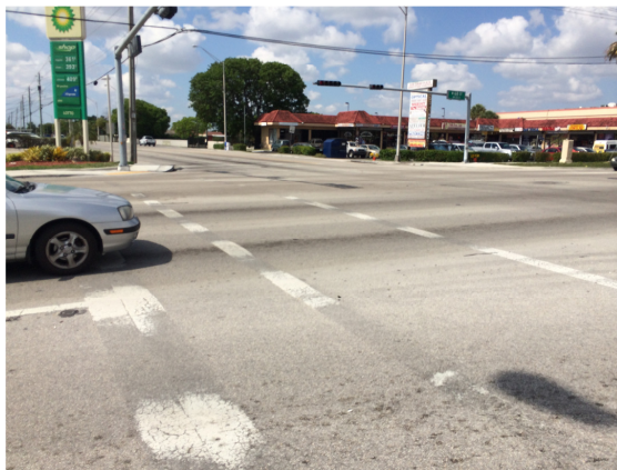
Faded pavement markings.
