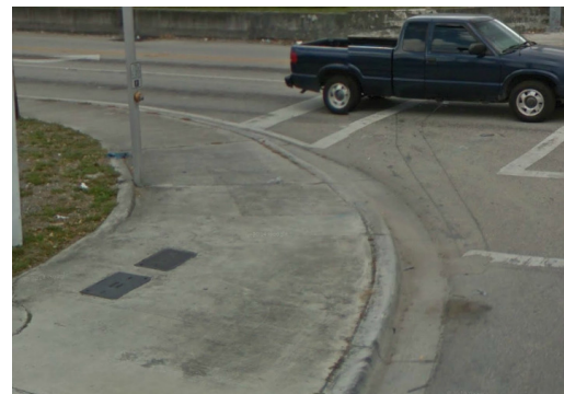
Pedestrian ramps are not ADA compliant at all corners.
