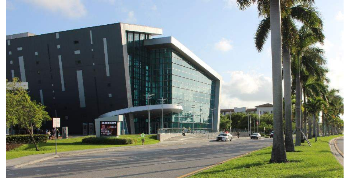
Figure 58: Existing conditions at SW 211 Street adjacent to Miami-Dade Cultural Arts Center
