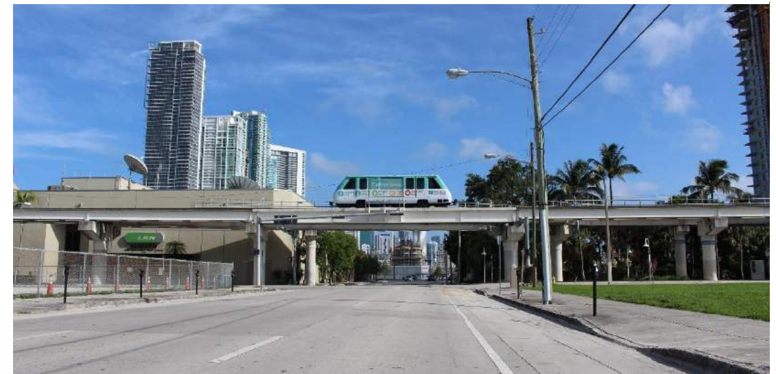
Figure 49: Existing conditions at North Miami Avenue and NE 15 th Street
