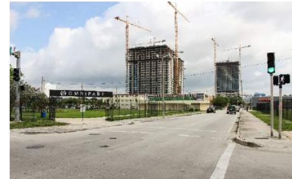
Figure 42: North Miami Avenue at NE 13 th Street
