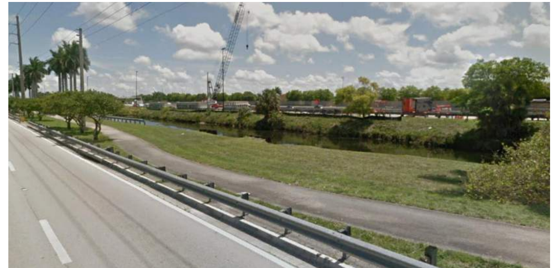
Figure 35: Snapper Creek; Image courtesy of Google Earth
