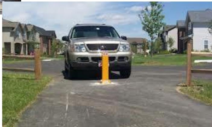
Use bollards to prevent motor vehicles from using the connection.
