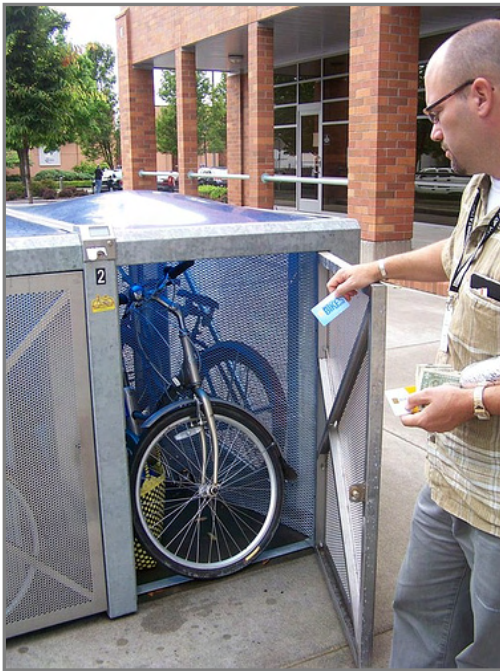
Inside View of a Bicycle Locker
