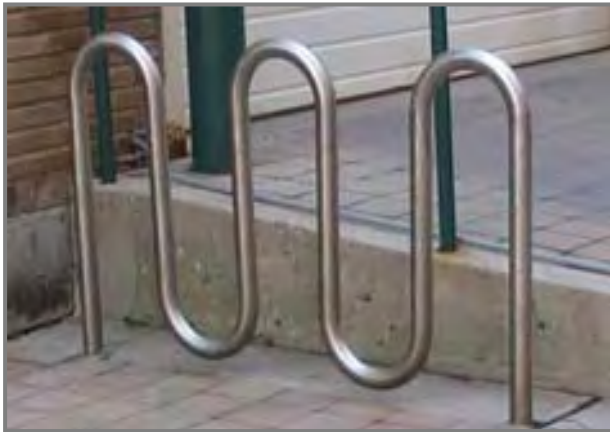
Serpentine rack too close to obstacles
