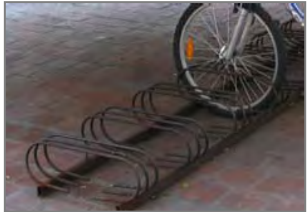
Rack with unstable support
