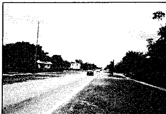
NE 15 th Avenue south of SR 826
