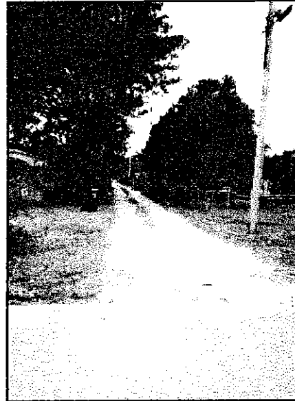
Existing alley, prior to reconstruction
