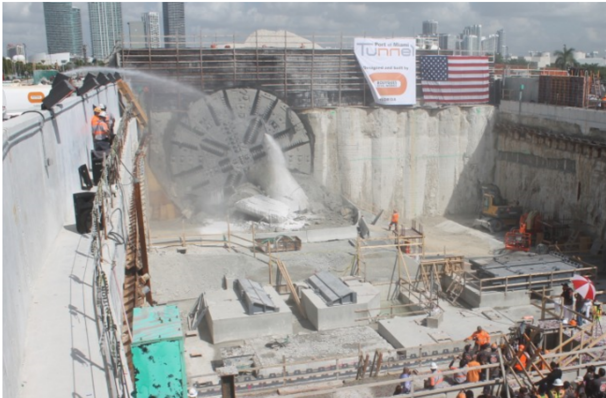
Figure 3-18 Breakthrough of First of Two PortMiami Tunnel Bores
