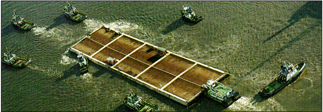
Figure 3-14 Immersed Tube Tunnel Section Being Transported to Site
