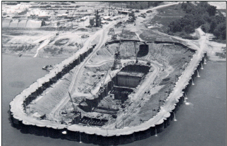
Figure 3-12 Cut and Cover Construction
