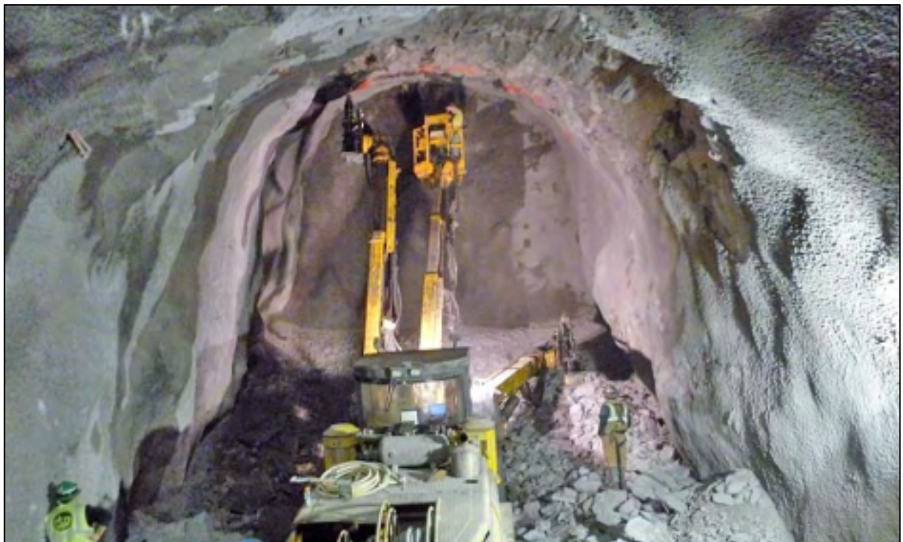
Figure 3-21 Tunnel Mining in the 2 nd Avenue Subway Project
