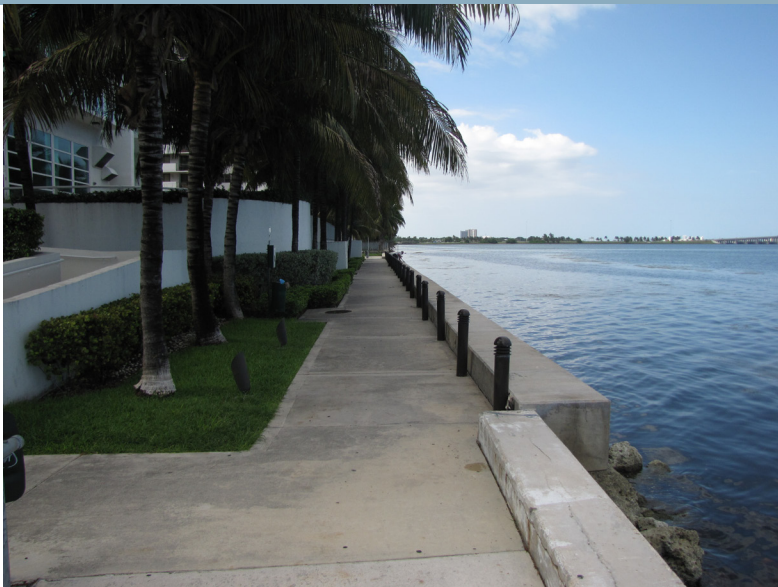
Completed bay side segment North of NE 25th Street. Segment is 6 feet wide, require widening to 8 feet.
