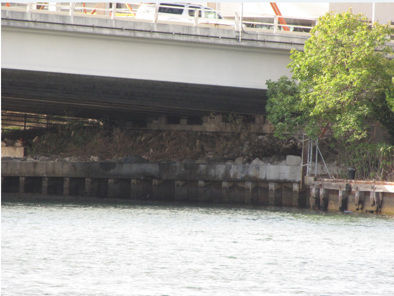
View looking Southwest at MacArthur Bridge (I-395). Existing bulkhead needs to be extended under bridge to create space for Baywalk.
