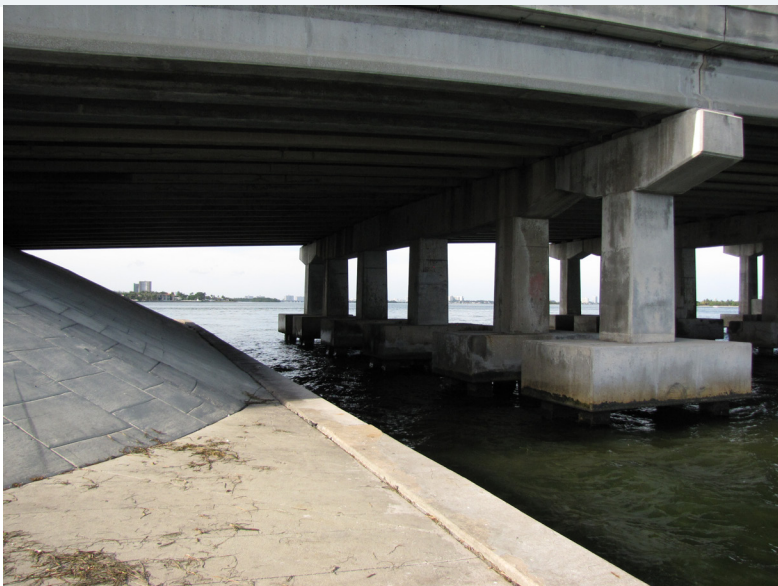
Julia Tuttle Causeway bridge abutment. Will need to remove sloped pavement to create a level access for shared path.
