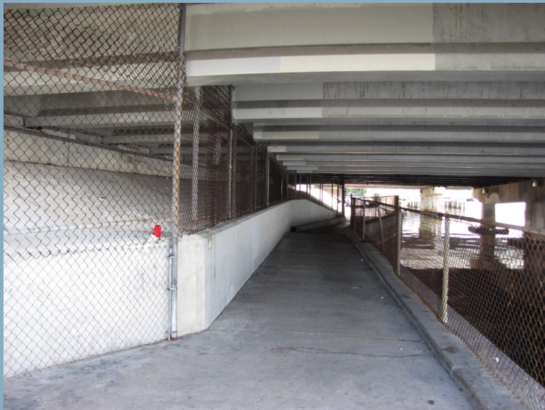
Existing bridge underpass at Rickenbacker Causeway. Width (7'-10") and height (8'-10") makes the space very tight and uninviting.
