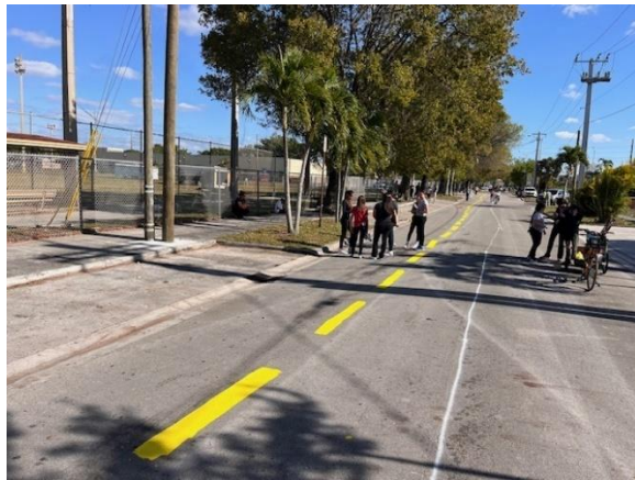
Figure 4- 24: Pavement markings on the pop-up bicycle lanes on W 6 Avenue.
