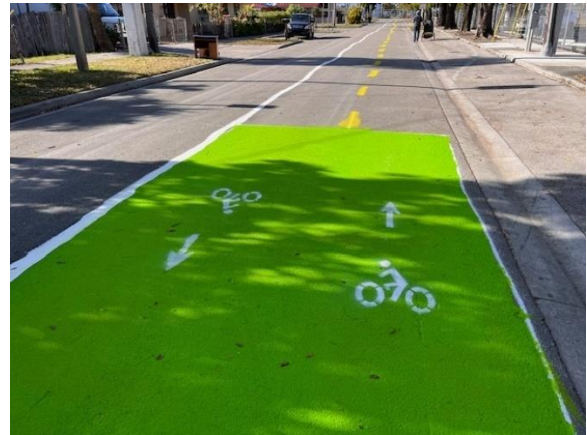
Figure 4- 26: Final layout of pavement markings to designate traffic flow separation on the pop-up bicycle lanes on W 6 Avenue.
