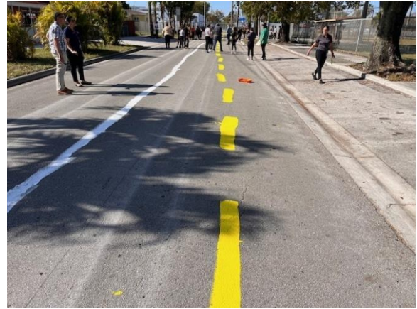
Figure 4- 25: Pavement markings for pop-up bicycle lanes on W 6 Avenue.
