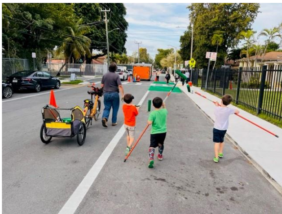
Figure 4- 10: Participants heading towards the beginning of the layout of the pop-up bicycle lanes to begin painting yellow pavement markings to designate bidirectionality on Matilda Street.
