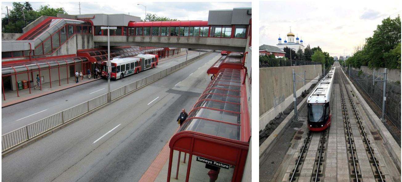
Figure 2 Confederation Line (Ottawa, CA) BRT to Rail Conversion Project Images
