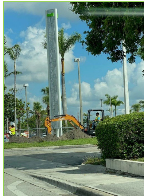
Figure 11 Ongoing Construction at the South Dade TransitWay Corridor Marlin Station
