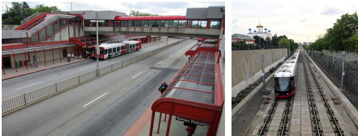
Figure 2 - Confederation Line (Ottawa, CA) BRT to Rail Conversion Project
