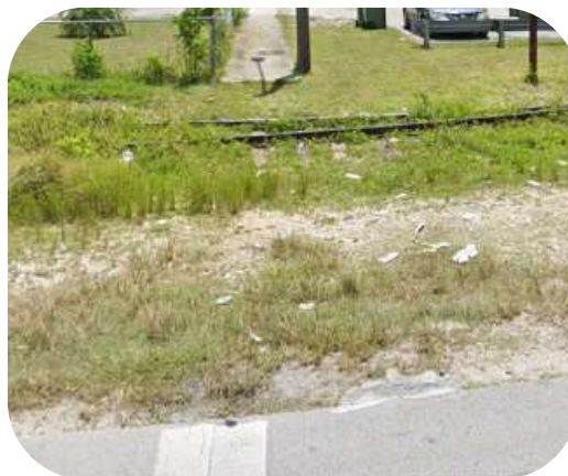
Example existing undermaintained CSX track connection in a school zone. Image Source: Google Streetview, 2022.
