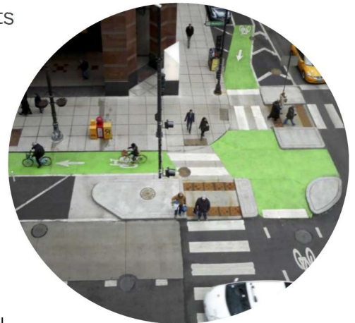
Corner of a protected intersection example, Looplink, Chicago, IL (Source: Flickr - John Greenfield.)
