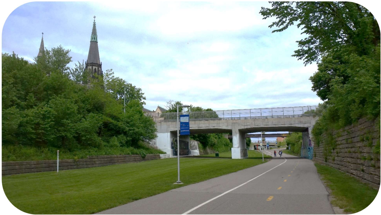
Dedicated future rail right-of-way on the left, with trail facilities on the right. Photo Source: Project team.
