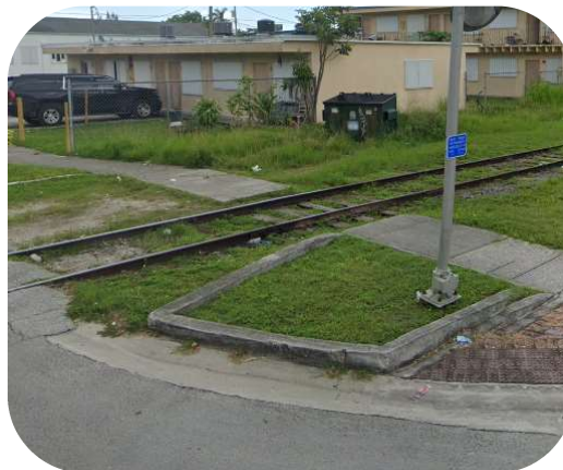
Example existing connection that could be improved at SW 4 th Street/10 th Avenue. Image Source: Google Streetview, 2022.
