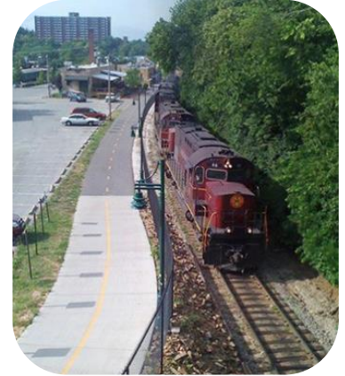
Frisco Trail in Arkansas with fencing, lighting, and narrow setbacks. Image Source: Rails with Trails: Best Practices and Lessons Learned .
