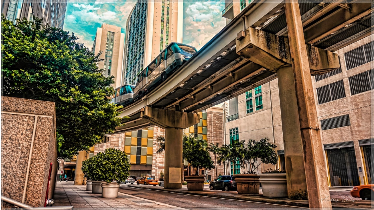
Figure 28. Column Supports for Two-Way Section – Existing Metromover System. Source: Flickr
