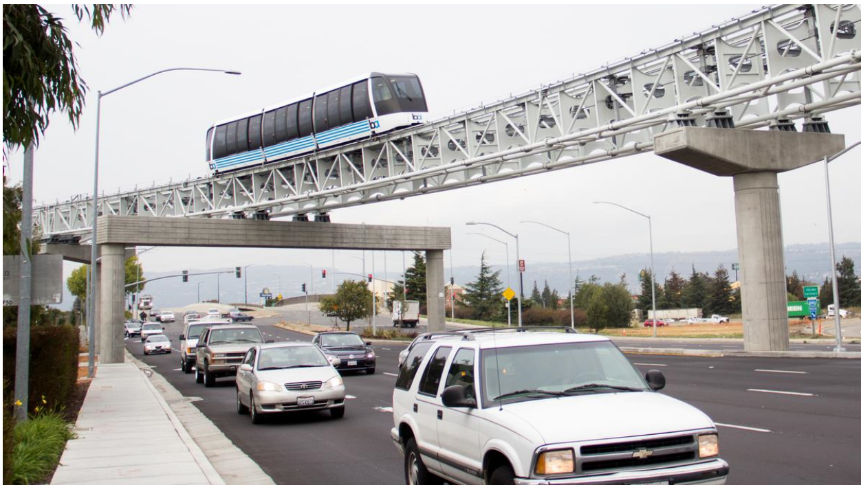
Figure 30. Column and Straddle Beam Supports for Oakland Airport Connector. Source: The Business Journals.
