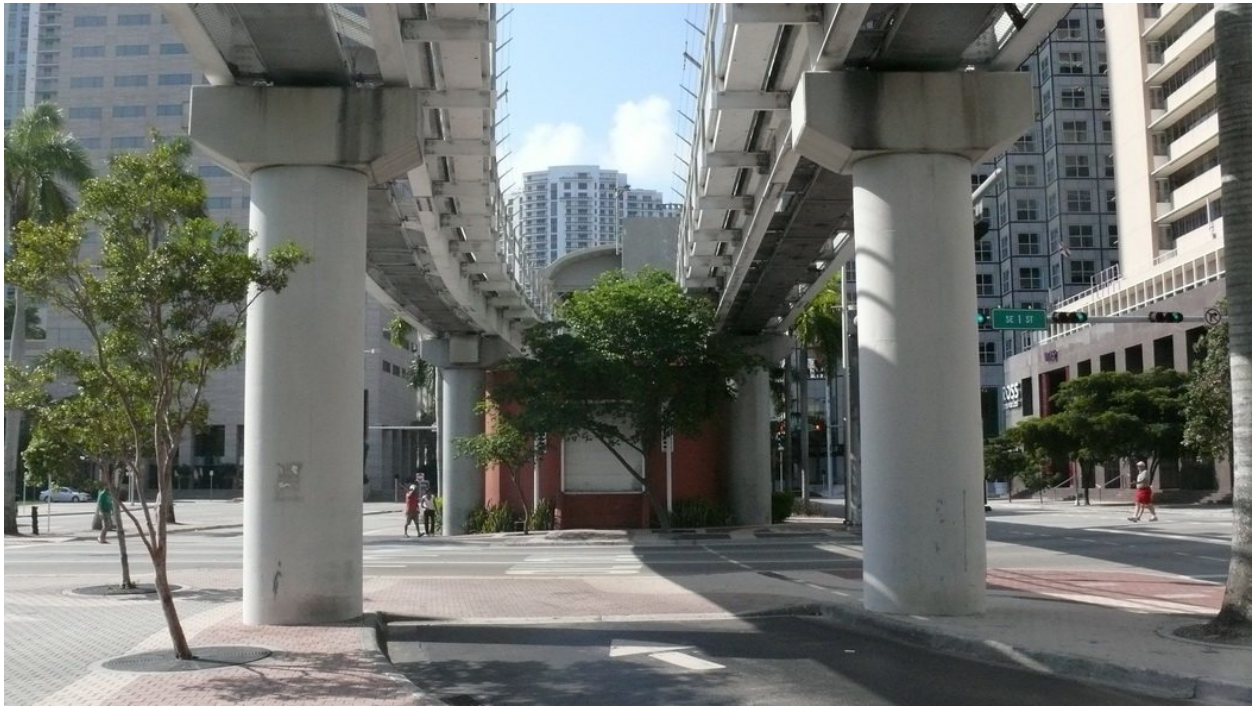
Figure 29. Column Supports and Guideway approaching a Station – Existing Metromover System. Source: frenchdistrict.com.
