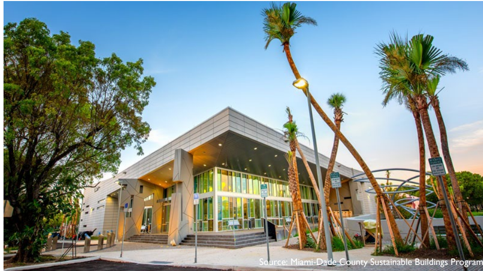
Figure 7: LEED-certified Aventura Branch Library
