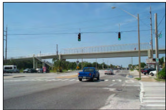
Typical Street Crossing Structure
