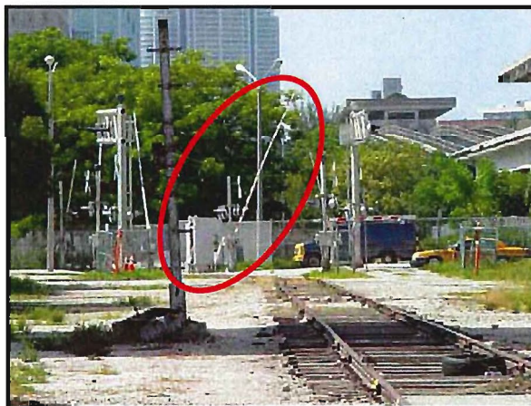
Exhibit 18: Crossing gate engaging yet no trains are approaching. This condition could result in severe delays.
