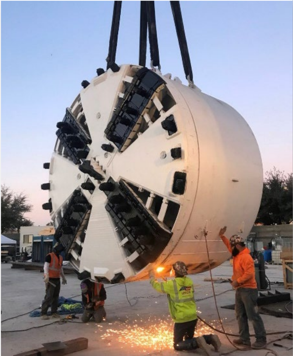
Figure 5: The frontal shield of the EPB transportation to the LVCC portal site (TBC, 2019)
