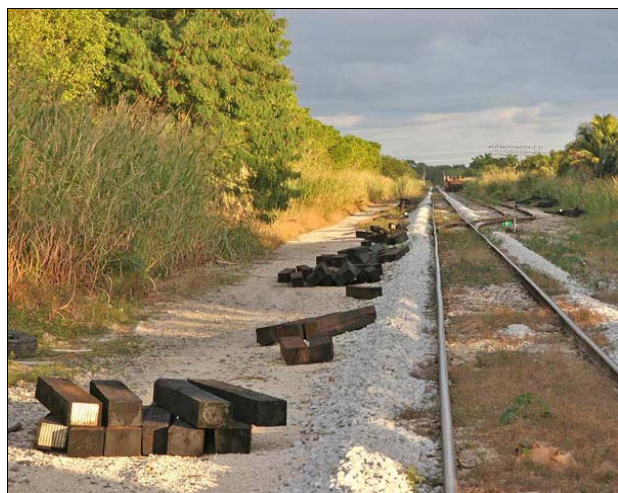
Exhibit 4.3 – Typical track, with new ties and ballast distributed for installation
