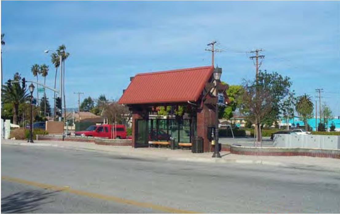
Bus Shelter Built Consistent with Architecture of Streetscaping Program and Pedestrian Lamps
