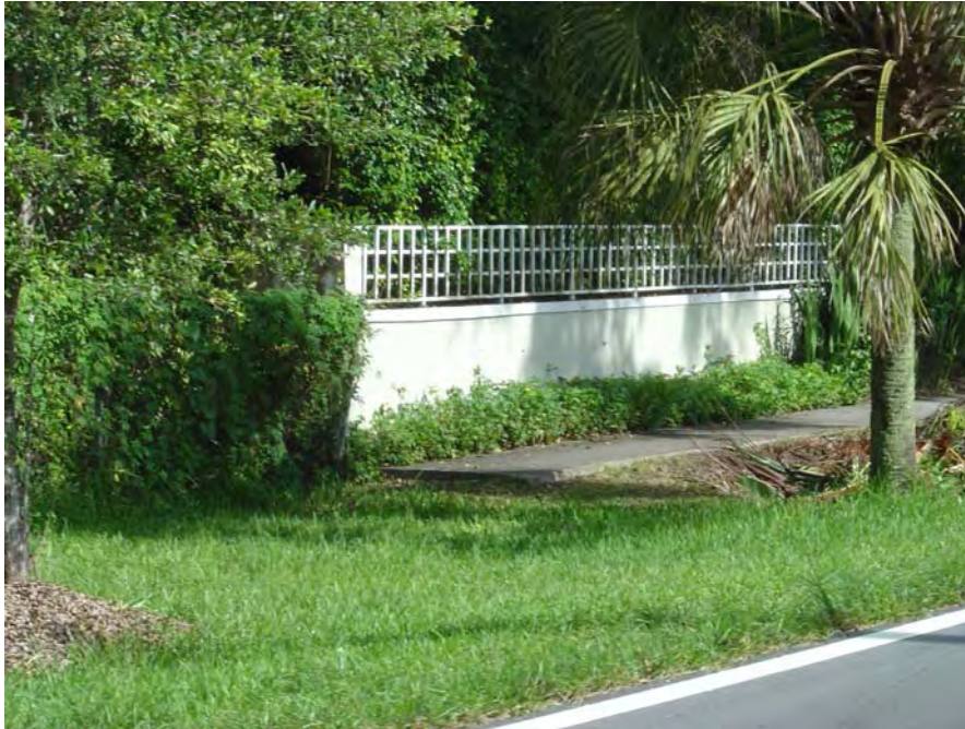
Exhibit 4. Discontinuous Sidewalk along Ludlam Road between Sunset Drive and Miller Drive
