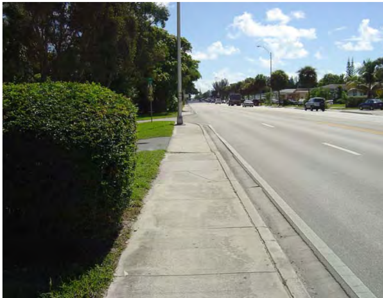
Exhibit 1. Typical Sidewalk Conditions along NW/NE 135 th Street
