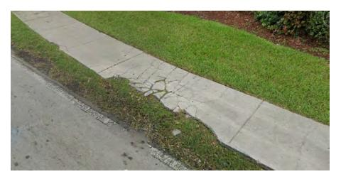
3. Reconstruct C&G and ramp to eliminate ponding issues
