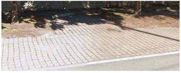
28. Repair sidewalk, Poses Tripping Hazard
