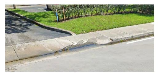
38. Propose Sidewalk Reconstruction. (Tripping Hazard)
