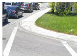
Missing detectable warning surfaces
