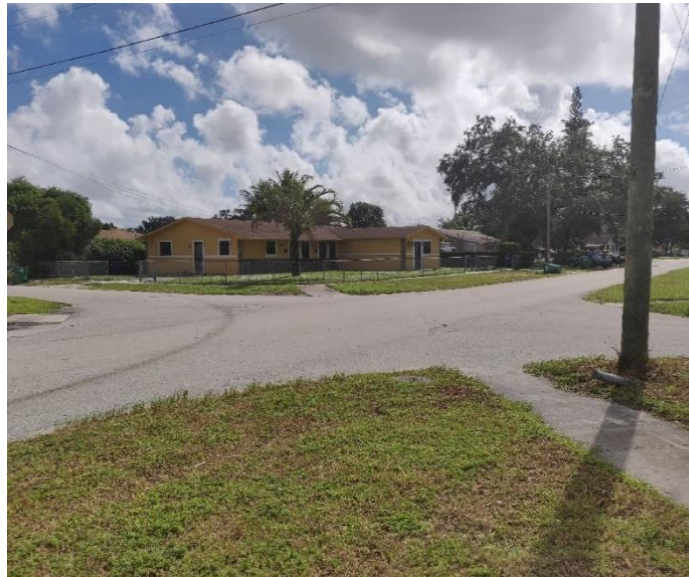
Missing crosswalks and ADA tactile surfaces
