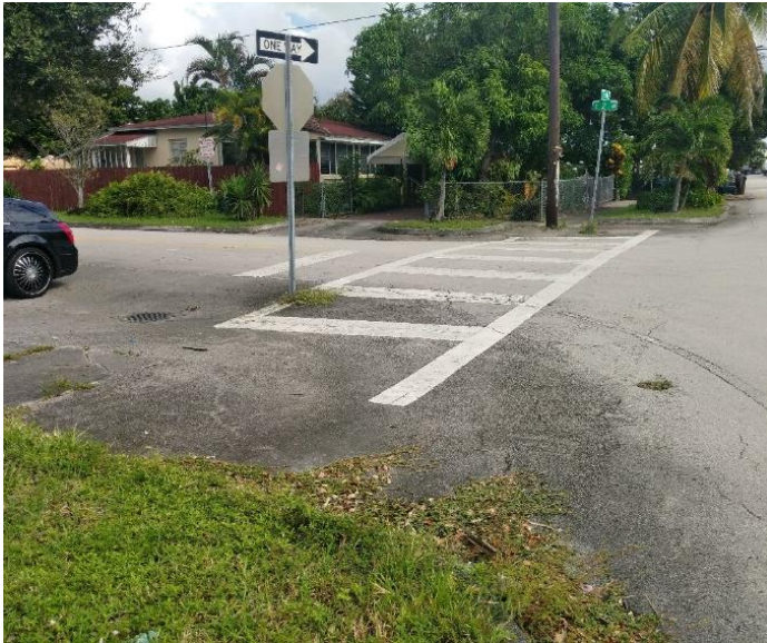
Missing sidewalk connection
