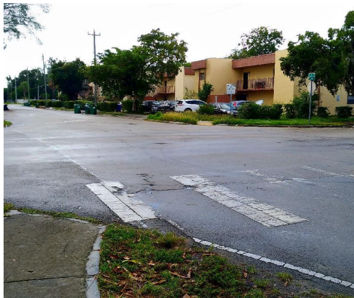
Crosswalk in need of restriping
