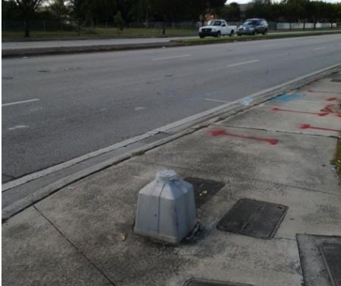
Pedestrian Push Button Pole Missing
