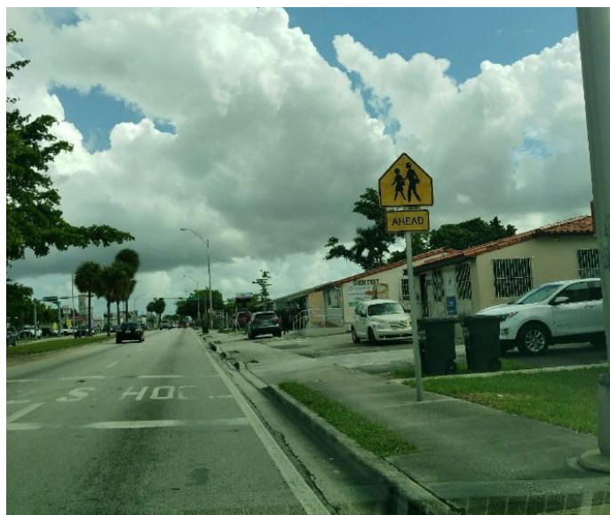
Faded Pavement Markings
