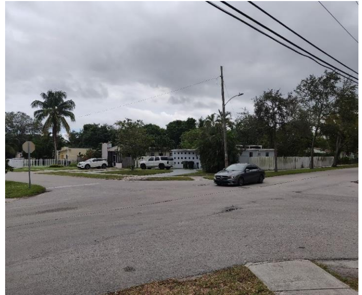
Missing detectable warning surface and crosswalks
