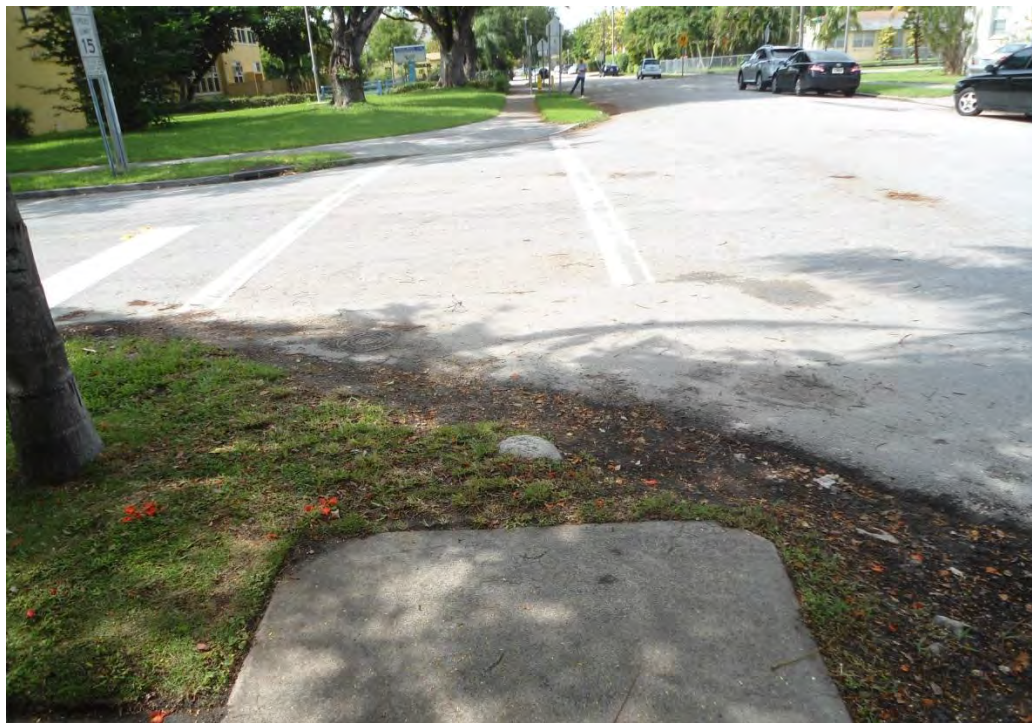
Provide access ramp connection and detectable warning pad
