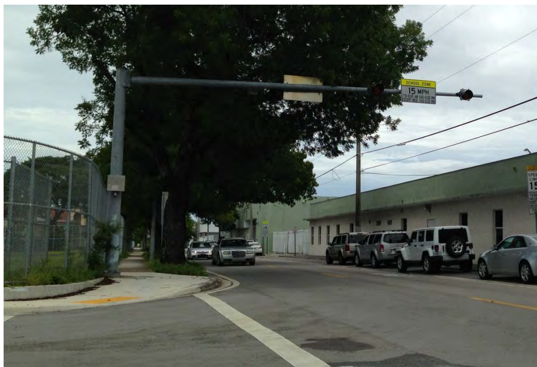
Replace sign panel on school zone assembly to read "15 mph school zone when flashing"
