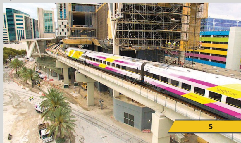
Brightline’s MiamiCentral Station Under Construction
