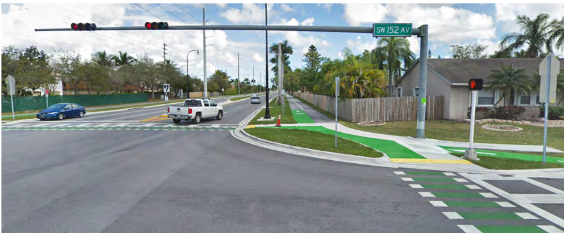
FIGURE 73 SW 152 ND STREET - "INTERESTED BUT CONCERNED" FACILITY
