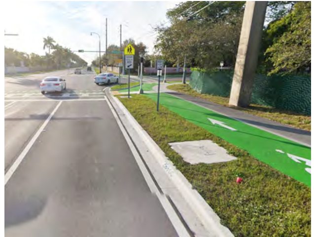
FIGURE 29 SEPARATED BIKE LANE SW 152 ND STREET, MIAMI, FL
