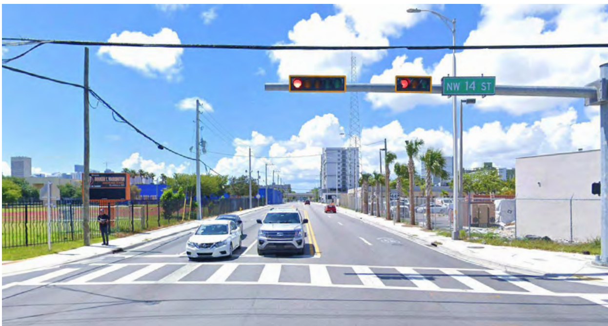
FIGURE 92 HIGH EMPHASIS CROSSWALKS AT SR 7/NW 7 TH AVENUE AND NW 14 TH STREET
