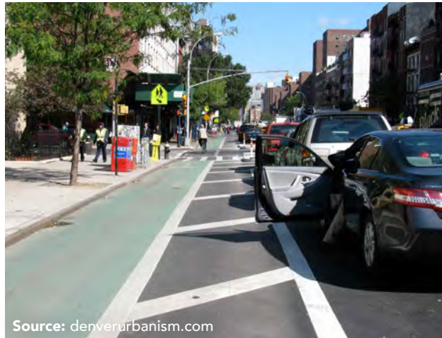
FIGURE 33 DENVER BUFFERED BIKE LANE
