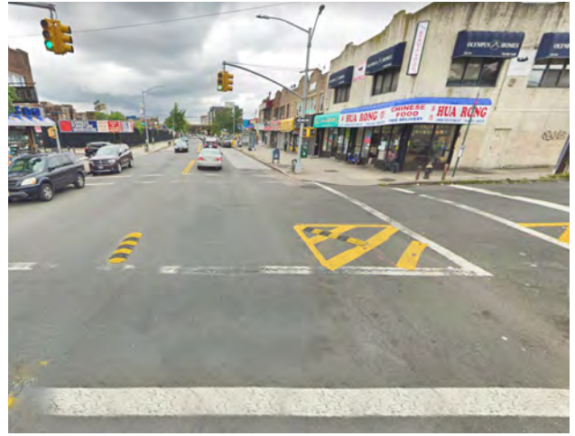
FIGURE 97 132 ND STREET & JAMAICA AVENUE TURNING WEDGE
