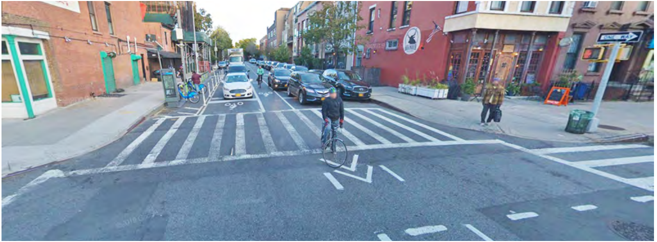
FIGURE 95 RECESSED STOP LINE - BERGEN STREET & VANDERBILT AVENUE NYC
