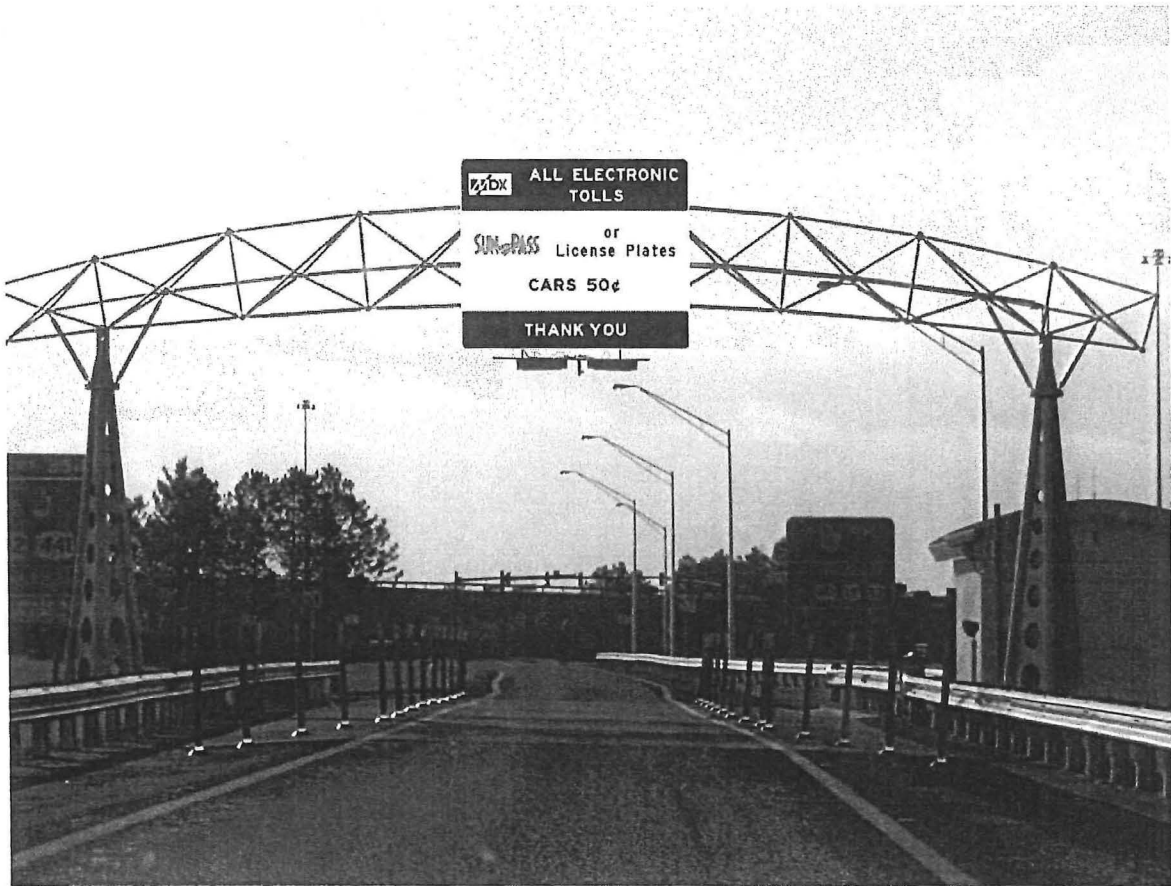
Figure 3-2 – Ramp Gantry with possible toll signing.
