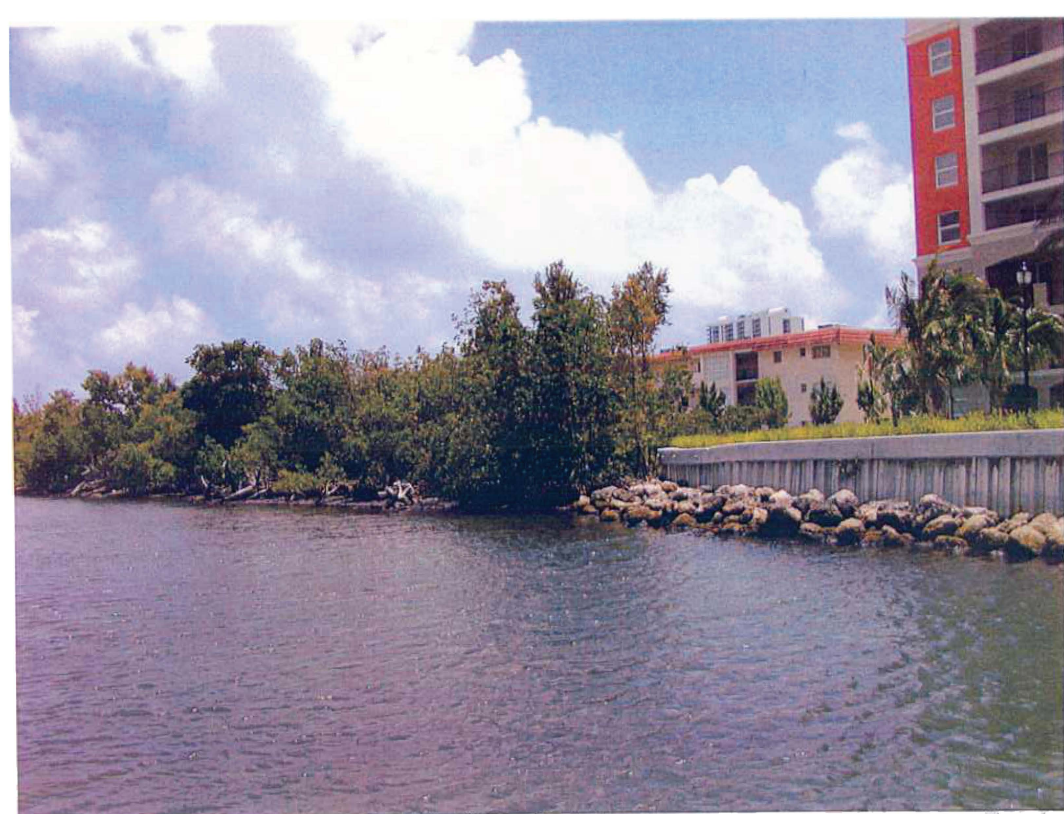
Looking ESE From Canal at Impact Area
