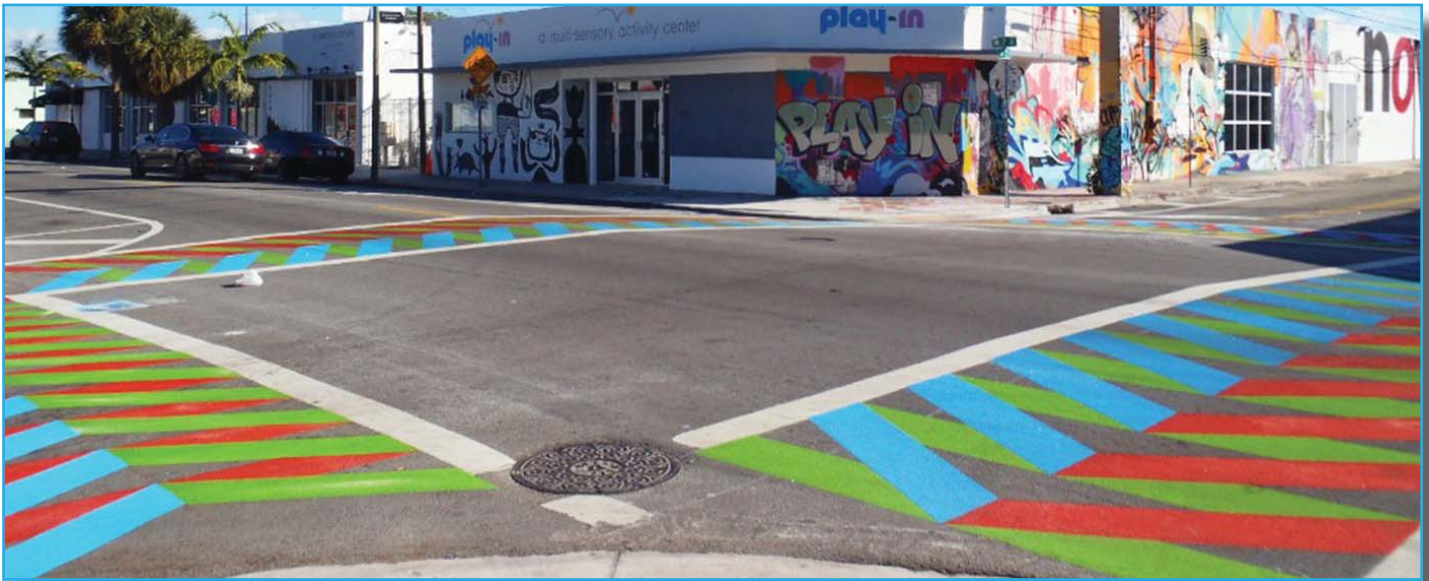
Sample "specialty paving treatment" on a city street
