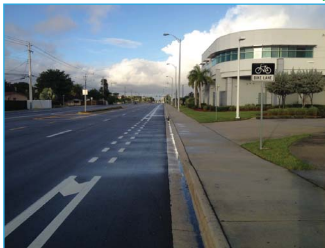
Sample “buffered bike lane” on a city street
