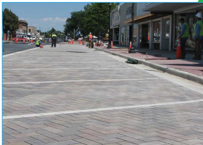
Sample “permeable pavers”
