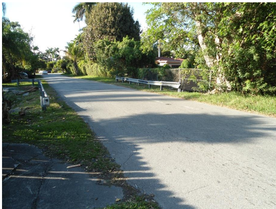
Absence of pedestrian facilities over a culvert
