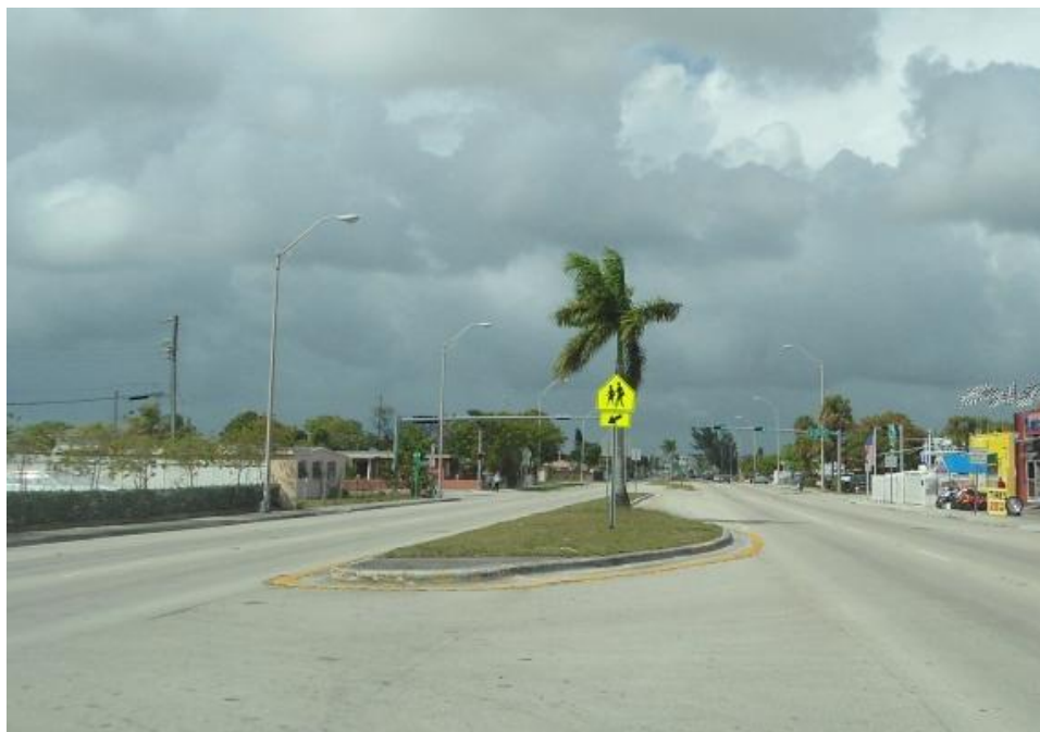
Incorrect advance school crossing sign
