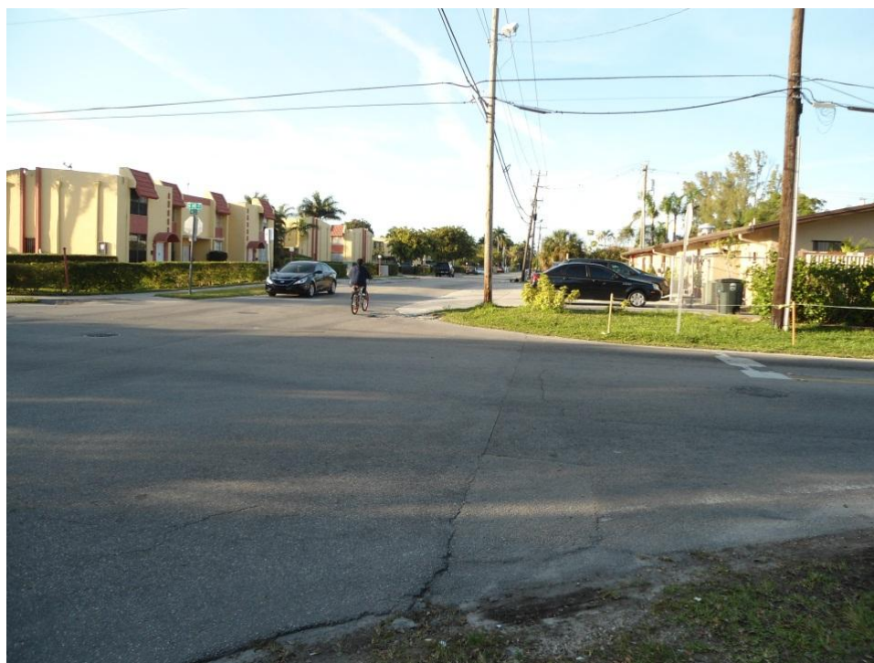
Absence of pedestrian crossing facilities
