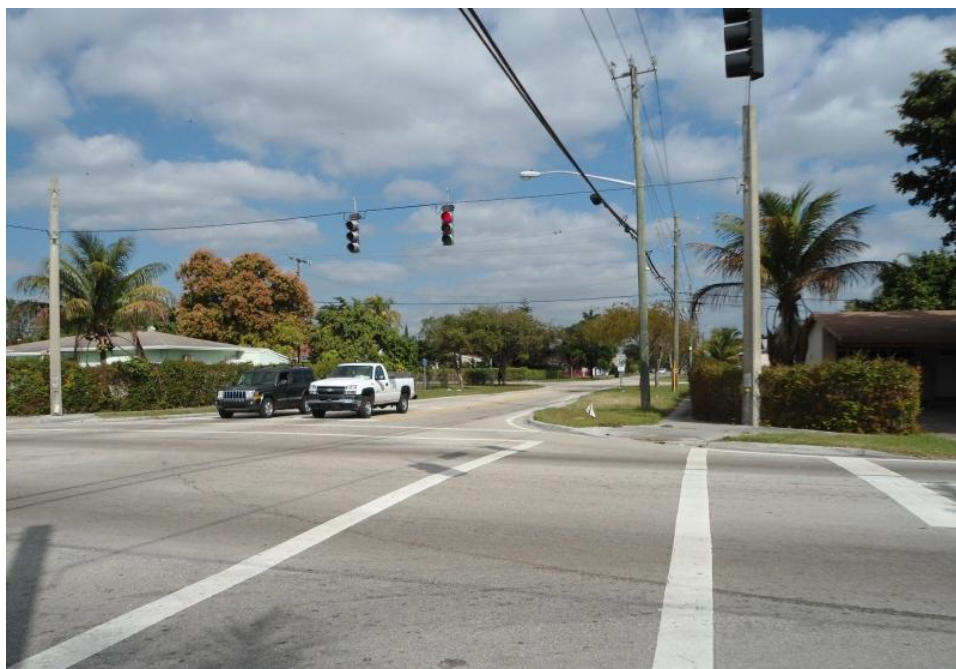
Signalized crosswalk without pedestrian signal displays
