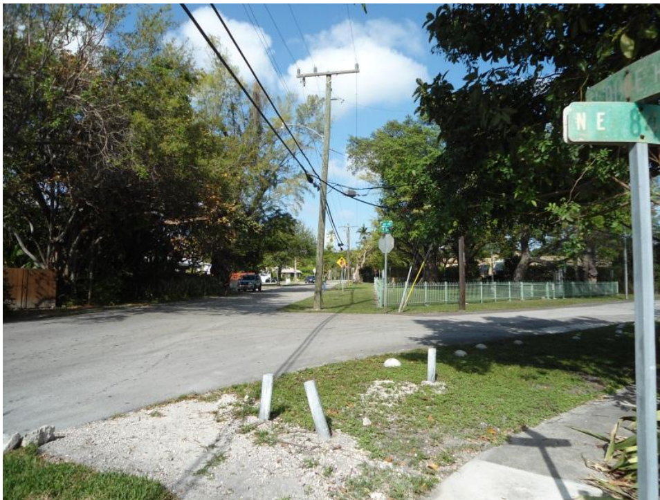
Absence of continuous sidewalk (and crosswalk)
