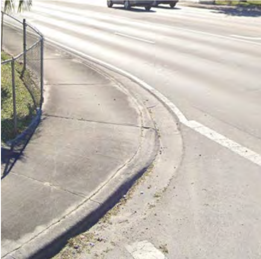
64. Install/ Replace Detectable Warning and Propose New Crosswalk Striping
