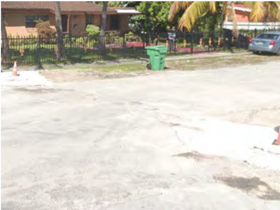
71. Install/ Replace Detectable Warning
