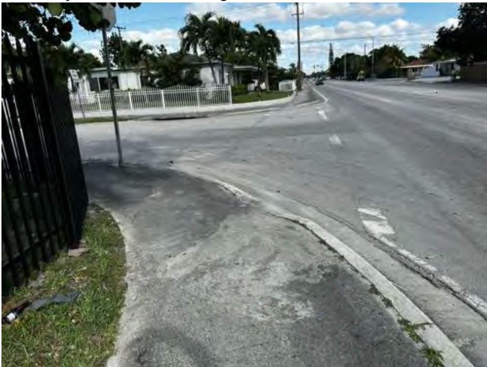
81. Install/ Replace Detectable Warning
