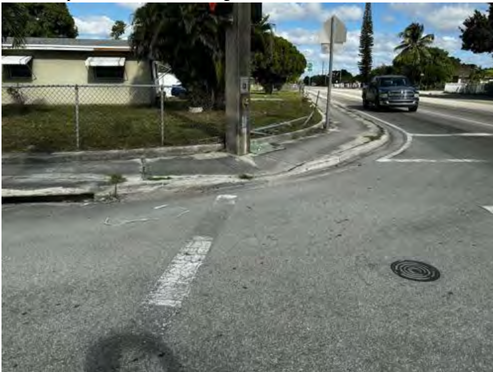
65. Install/ Replace Detectable Warning
