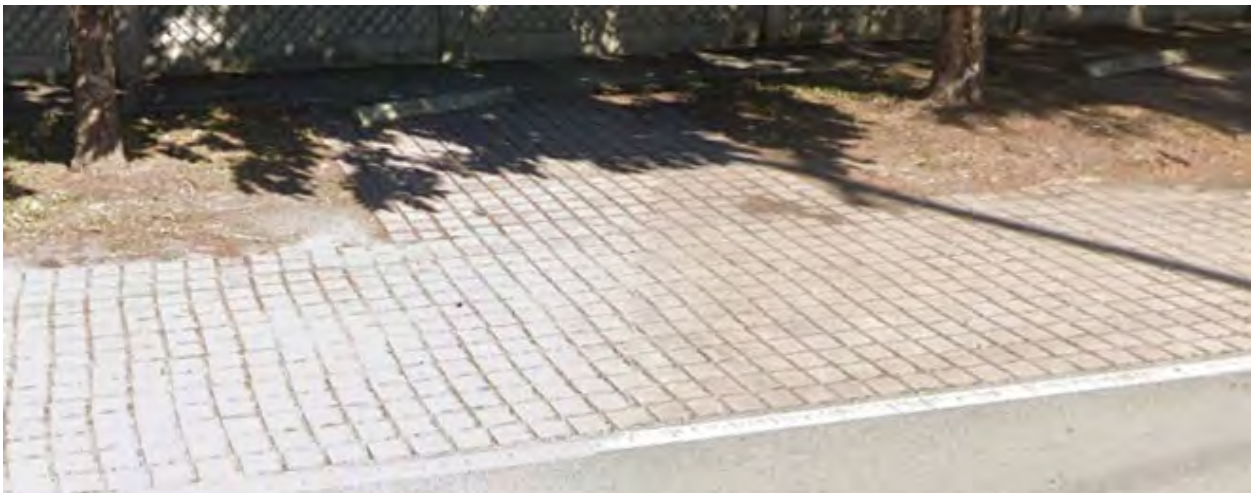
27. Repair sidewalk, Poses Tripping Hazard
