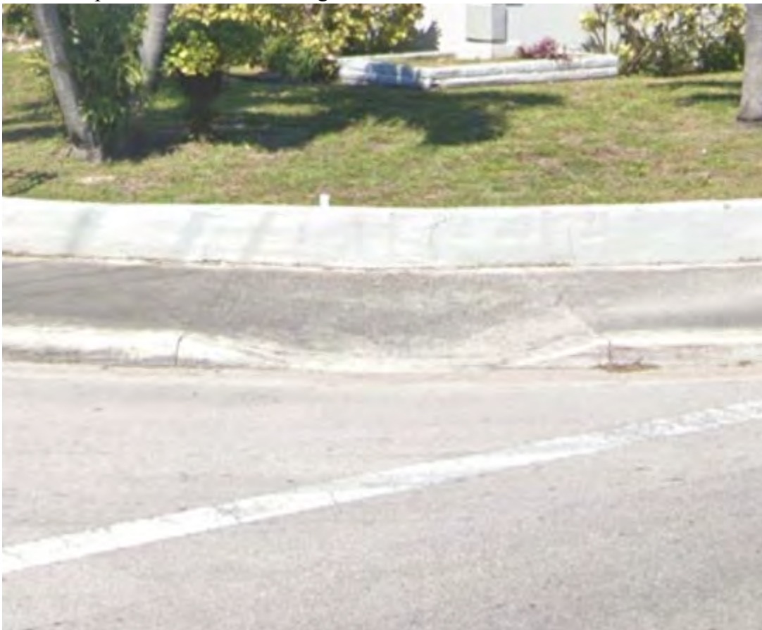
79. Install/ Replace Detectable Warning
