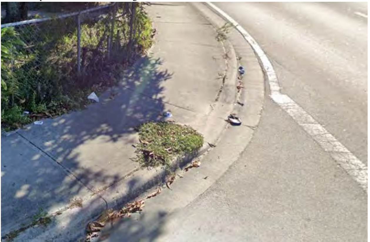
15. Install/ Replace Detectable Warning
