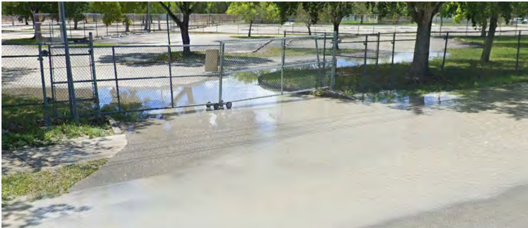
26. Install Detectable Warnings at curb ramps
