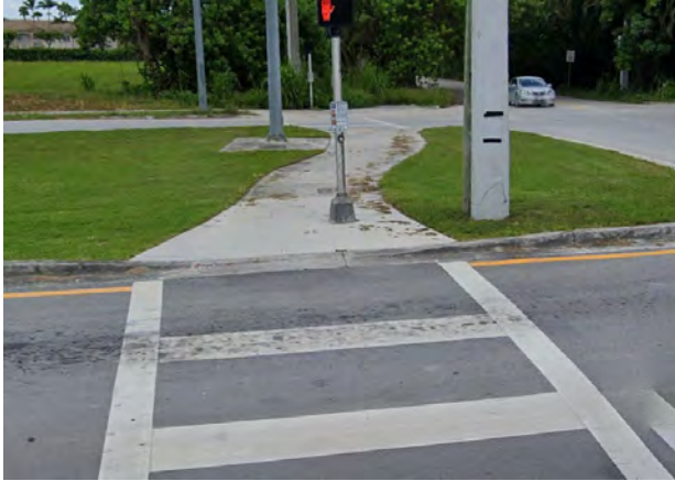
22. Remove Existing Sign
