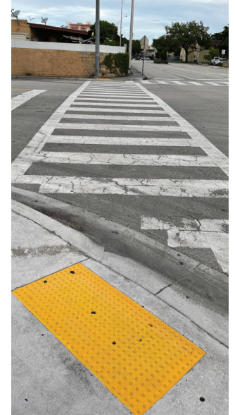
Crosswalk with ADA Feature
