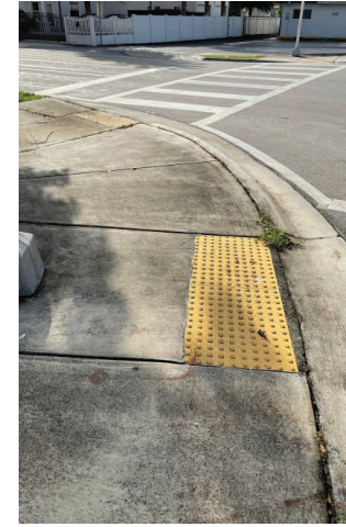
Crosswalk with ADA Feature
