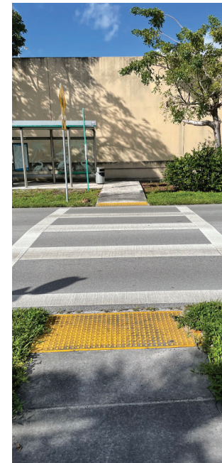
Crosswalk with ADA Feature
