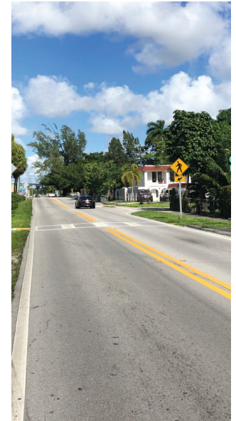
Pedestrian Crossing Signage
