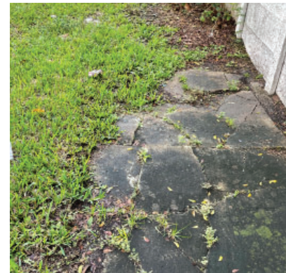
Damaged Pavement
