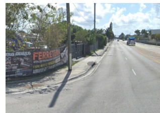
Utility pole obstruction in sidewalk
