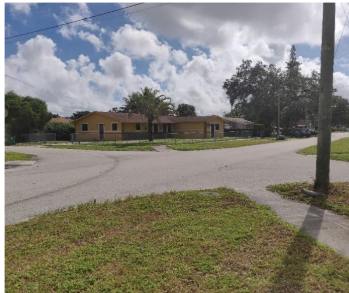
Missing crosswalks and ADA tactile surfaces
