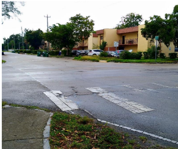
Crosswalk in need of restriping
