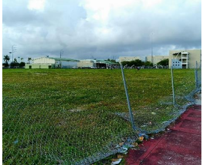
School Fence in Disrepair
