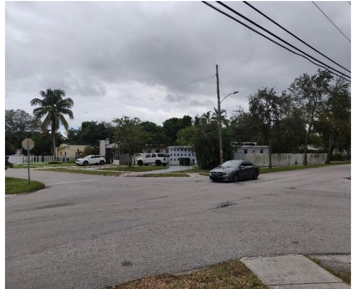
Missing detectable warning surface and crosswalks
