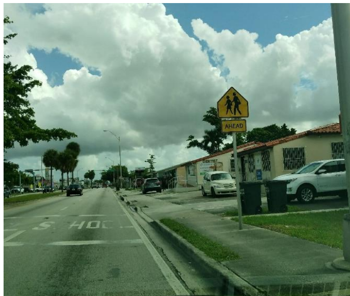
Faded Pavement Markings
