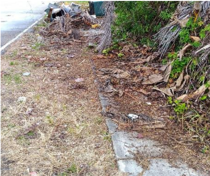
Debris Impeding Sidewalk Access
