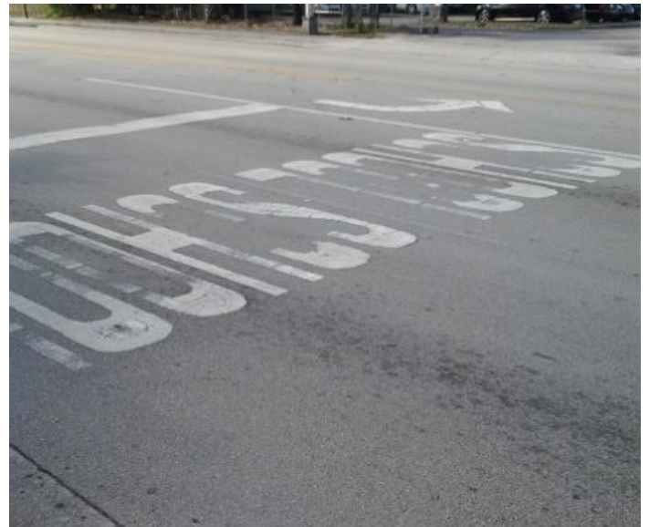
Restripe Pavement Markings
