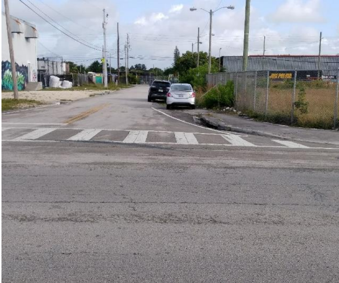
Install Tactile surfaces
