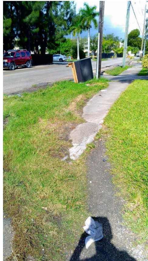
Overgrown vegetation impeding sidewalk
