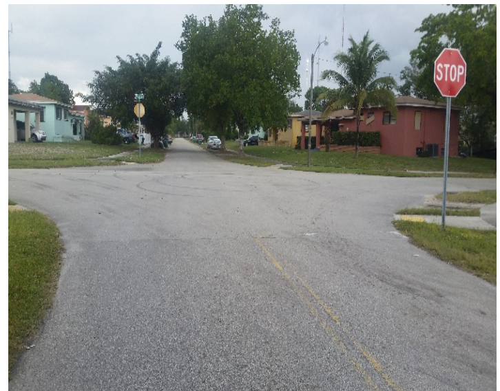
Faded pavement markings
