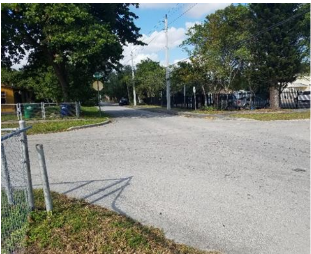
Figure 61: Lack of Sidewalks and Crosswalks
