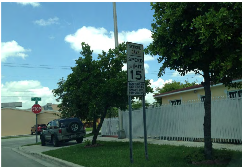
Refurbish worn school speed zone sign
