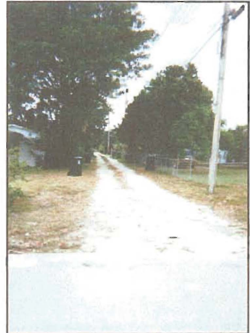
Existing alley, prior to reconstruction
