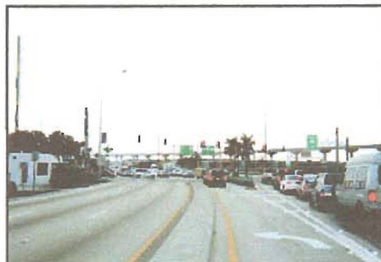
SR 826 westbound towards Golden Glades Interchange
