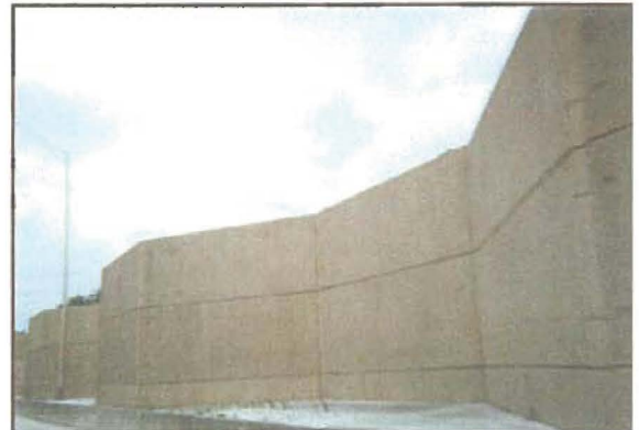
Existing I-95 noise mitigation wall, near Aventura exit
