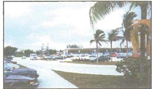
Existing Golden Glades Park and Ride Facility, near Tri-Rail Station
