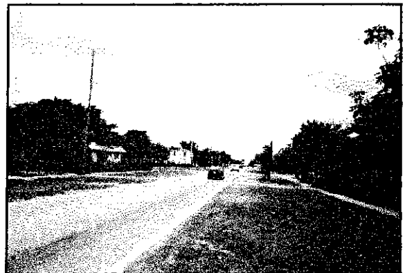
NE 15 th Avenue south of SR 826
