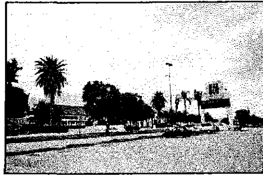
Mall at 163 rd Street, near proposed Mall Intersection
