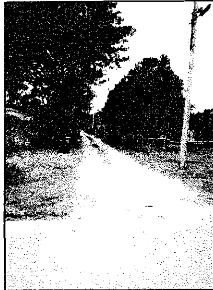
Existing alley, prior to reconstruction
