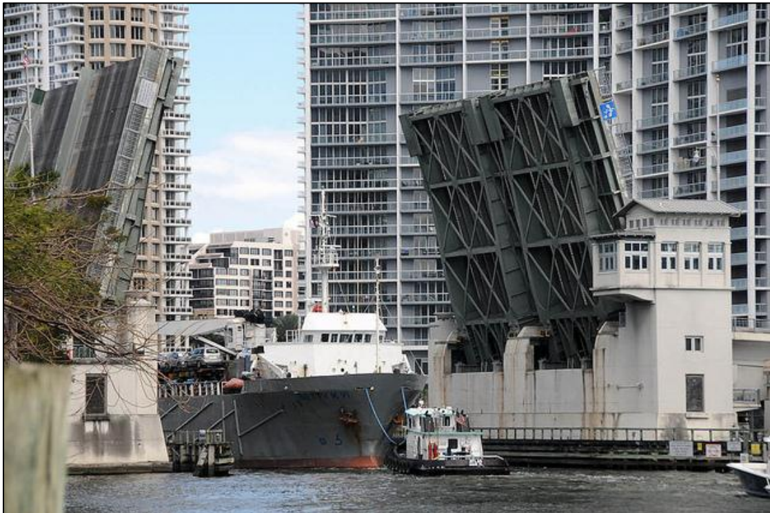
Figure 38: SW 2 Avenue Bridge
