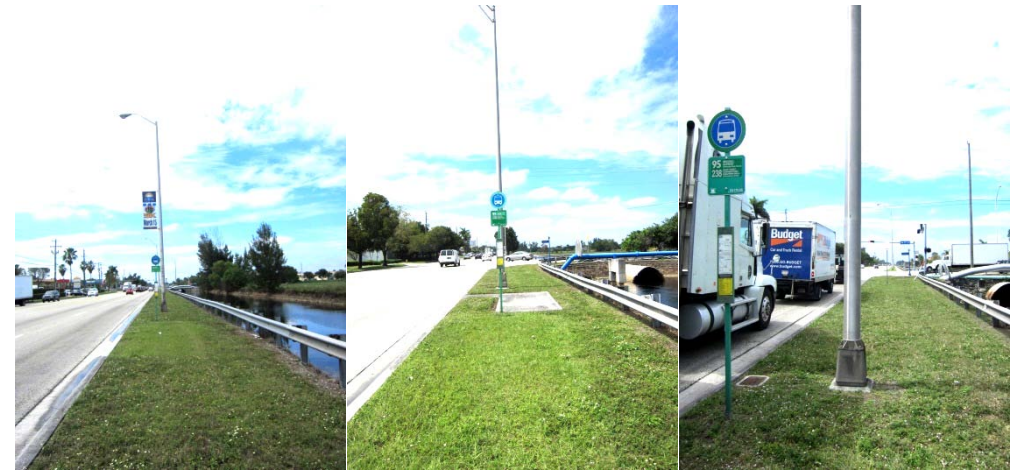
While these stops on NW 25 th Street in Doral are somewhat accessible, transit riders have to walk across long areas of uneven grass to reach them or disembark from them. As there are no landing pads, nor connected sidewalks, these stops are non ADA compliant.
