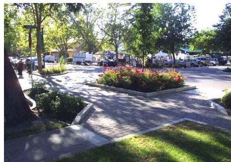
Bulbouts are curb extensions which can serve as neckdowns for traffic, and can be utilized to shorten crossing distances for pedestrians (Columbus, OH - Top Right). With innovation, they can also provide a rest area in a mini park, where people can sit (Keene, NH - Top Left), and city beautification, making walking a more enjoyable experience (Davis, CA - Bottom Left). Source: http://contextsensitivesolutions.org/
