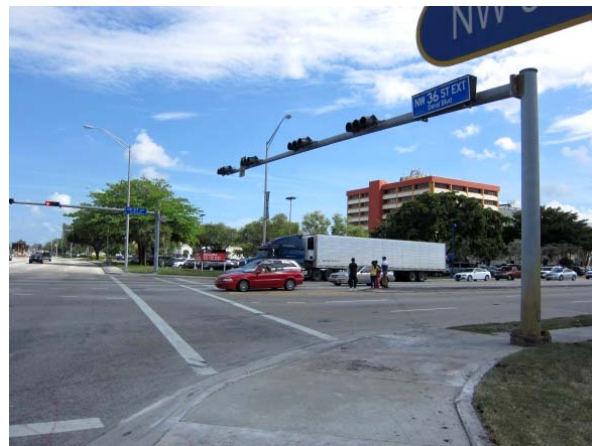
A family waits by the median as they were not able to complete their crossing in one cycle. Here, the family has moved from the crosswalk to the raised median in order to avoid being in the path of turning vehicles. The addition of a pedestrian island area would have reduced the exposure of the family to oncoming traffic.
