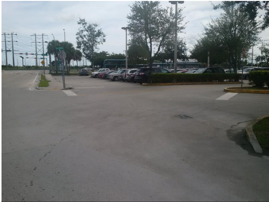
Entry/Exit point of the SW 244 th Street Park-and-Ride facility
