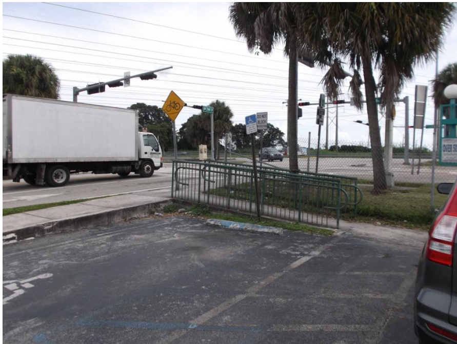
ADA Deficient sidewalk that requires a handrail
