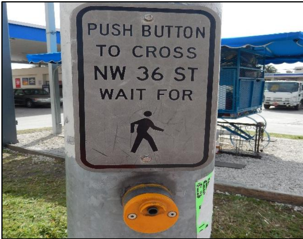
Photograph 10: Missing pedestrian push button on the southeast corner
