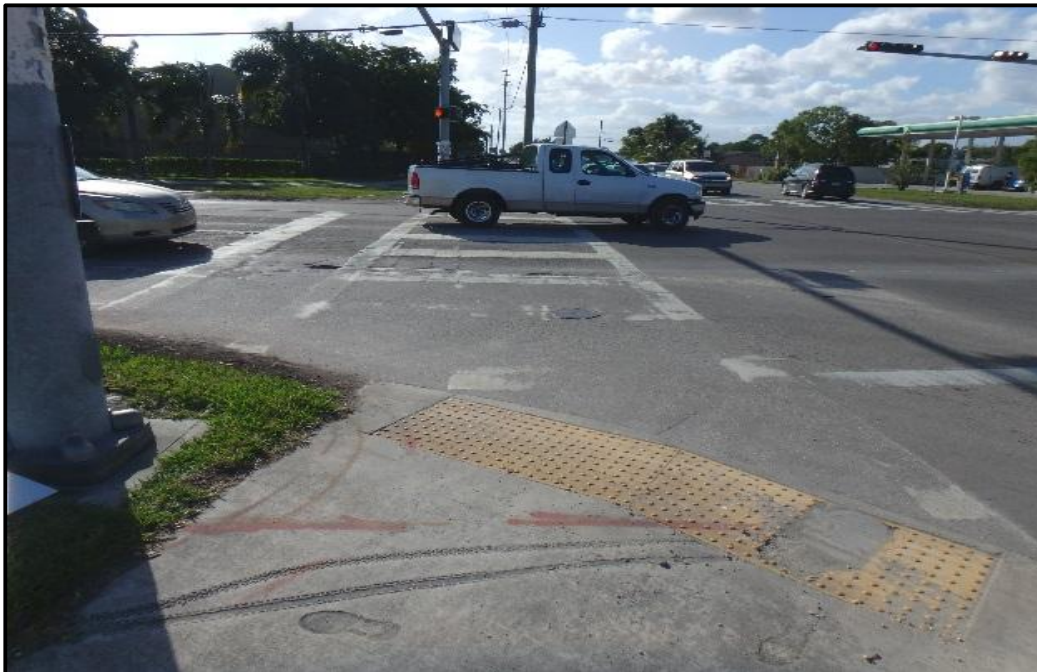
Photograph 21: Deficient pedestrian facilities
