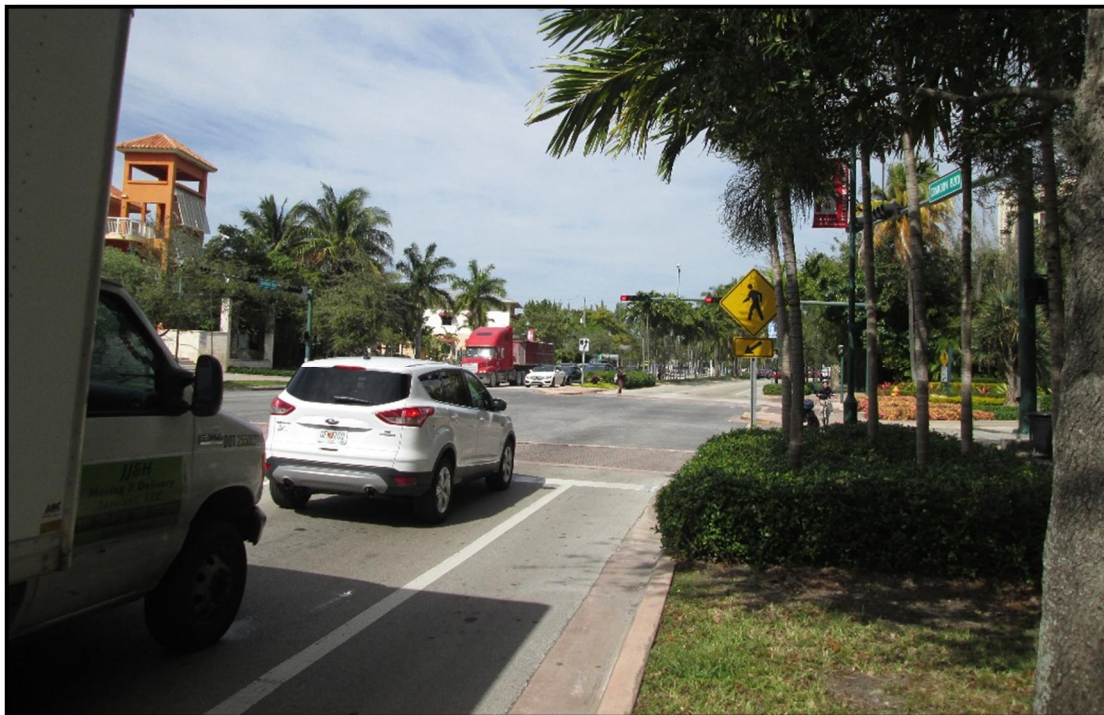
Photograph 32: Poor visibility of crosswalk for right-turning vehicles at Key Colony (looking north)
