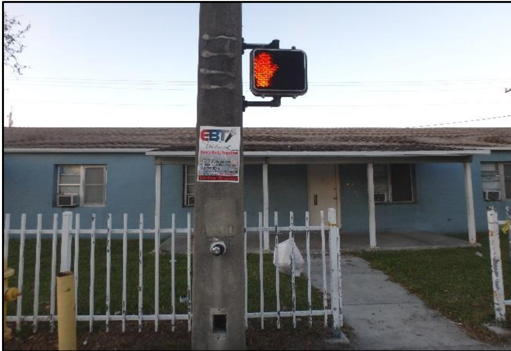
Photograph 15: Missing pedestrian signage at pedestrian signal east of NW 13 Court
