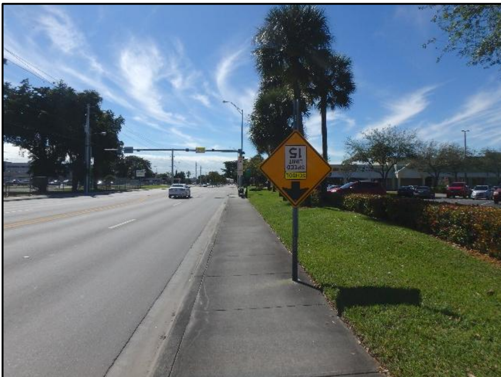
Photograph 23: Upside down school speed limit sign on the west side of south leg
