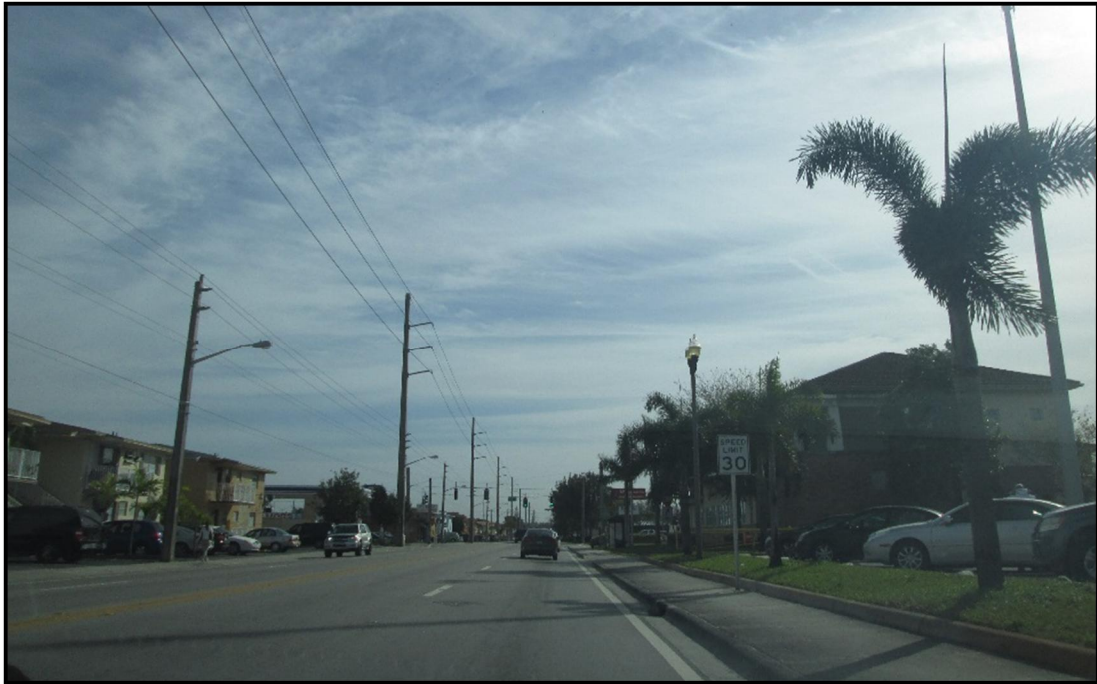
Photograph 40: View of W 29 Street corridor
