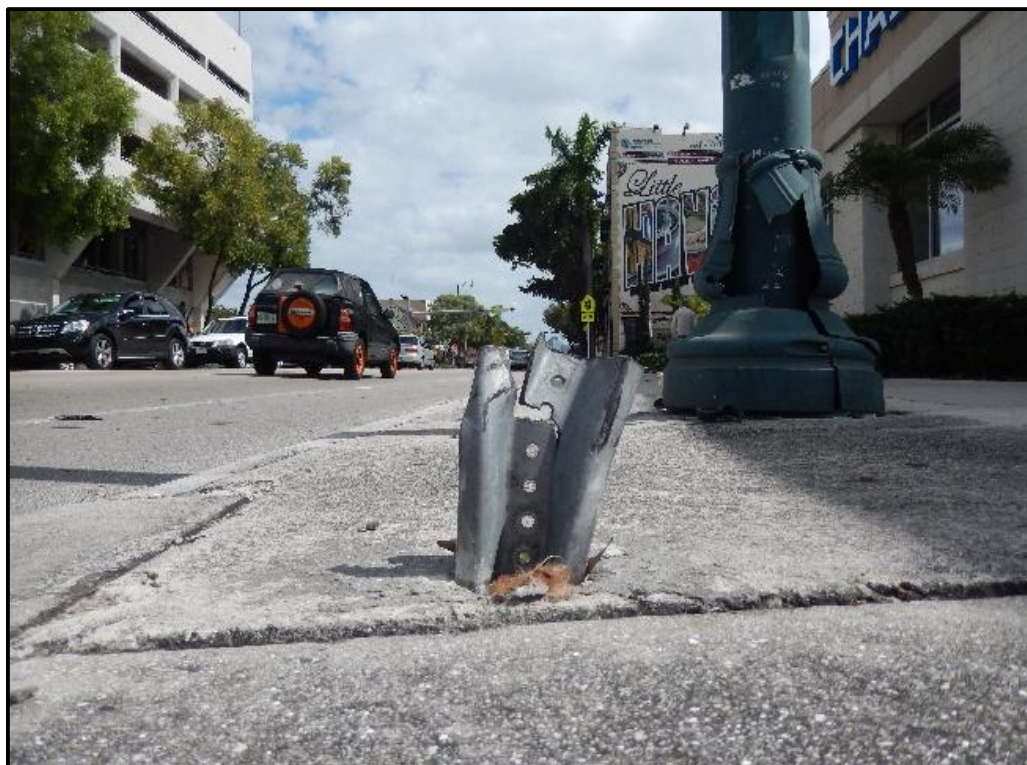
Photograph 7: Damaged sign post at the southeast corner
