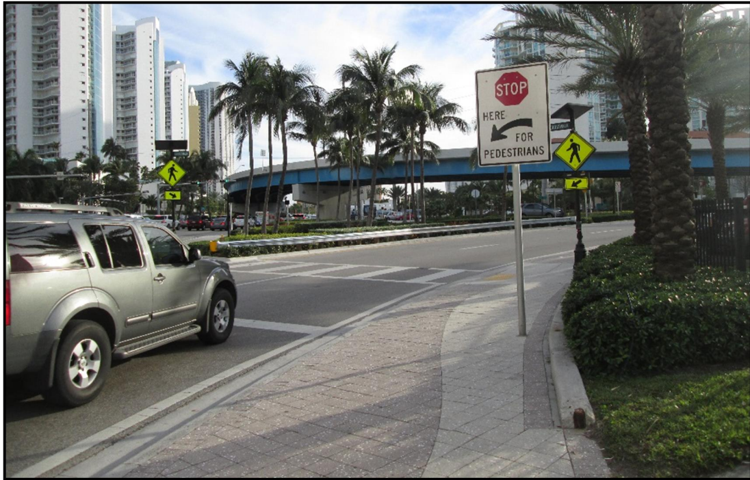
Photograph 37: Signage and RRFB at interchange of NE 163 Street and Collins Avenue
