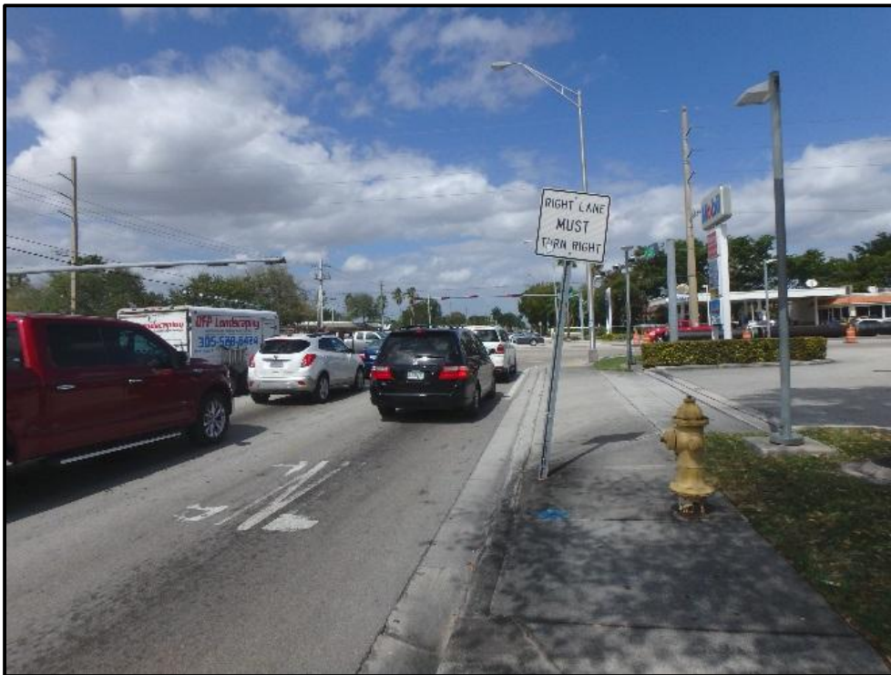
Photograph 19: Tilted sign for the northbound approach (too close to travel lanes)
