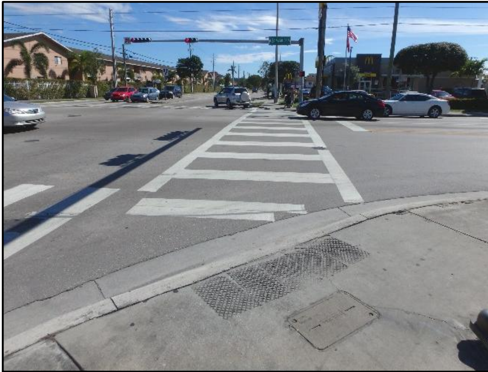
Photograph 22: Existing detectable warning surfaces
