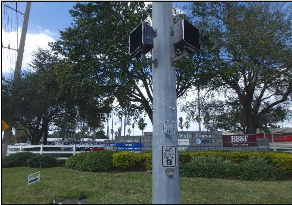
Photograph 18: Pedestrian push buttons and signage
