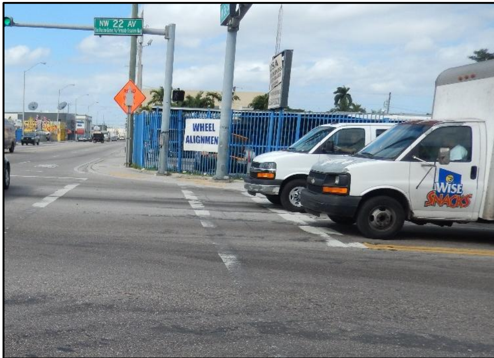
Photograph 12: Worn pavement markings and dim pedestrian walk indication
