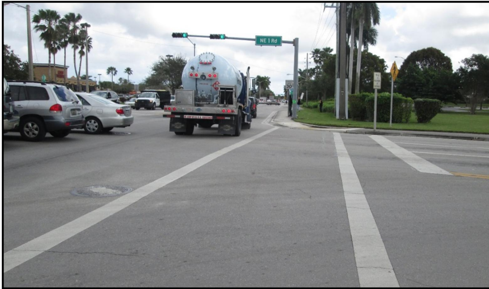
Photograph 59: No pedestrian signal displays for crossing at NE 1 Road
