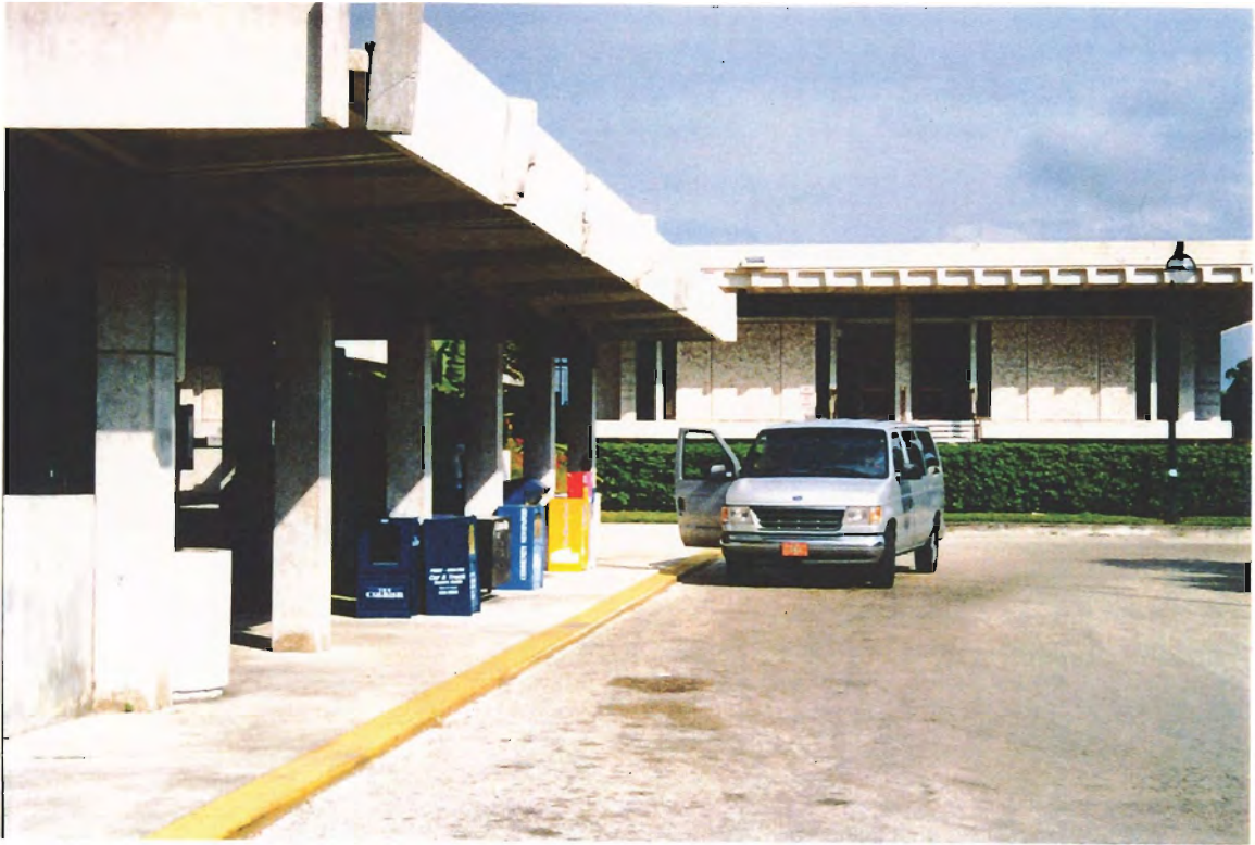
Bus stop (viewed from west).
