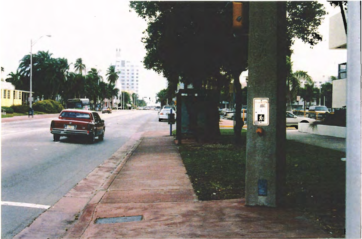
East side view of existing bus stop/proposed Intermodal Center bus bay.
