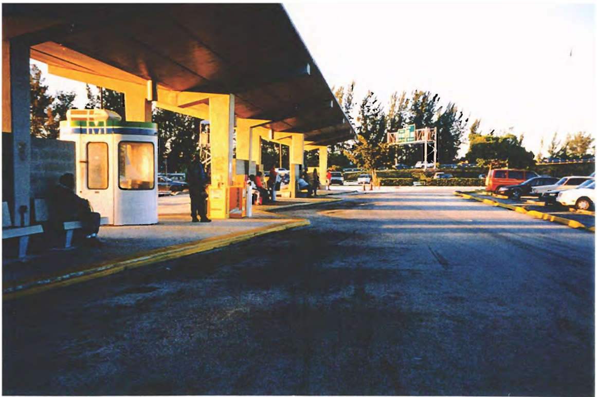
North view of bus terminal.
