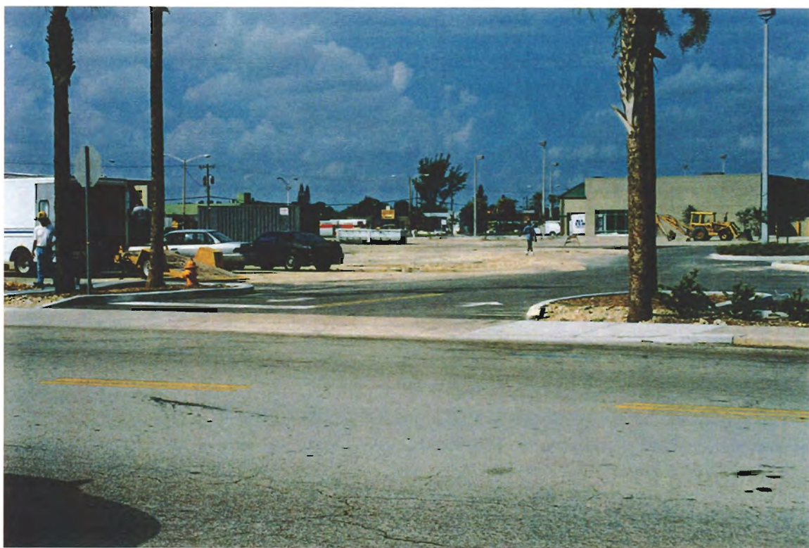
View of the driveway to the terminal's parking lot from 7th Avenue.
