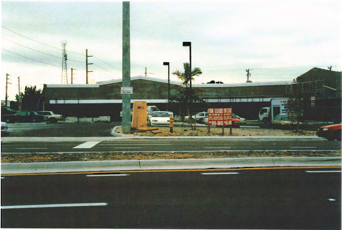
Parking lot on southwest side of US 1/163rd Street.
