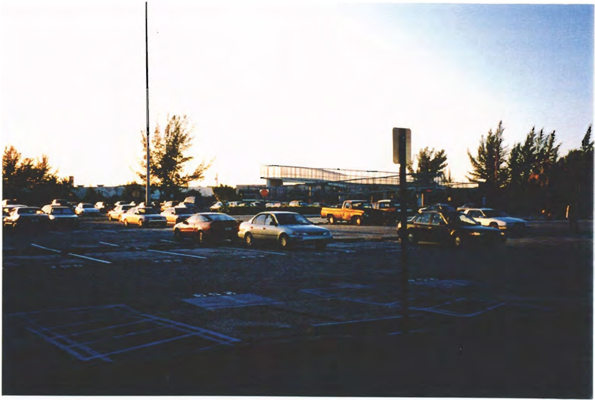
Northeast side view of Park-n-Ride lot and pedestrian overpass.
