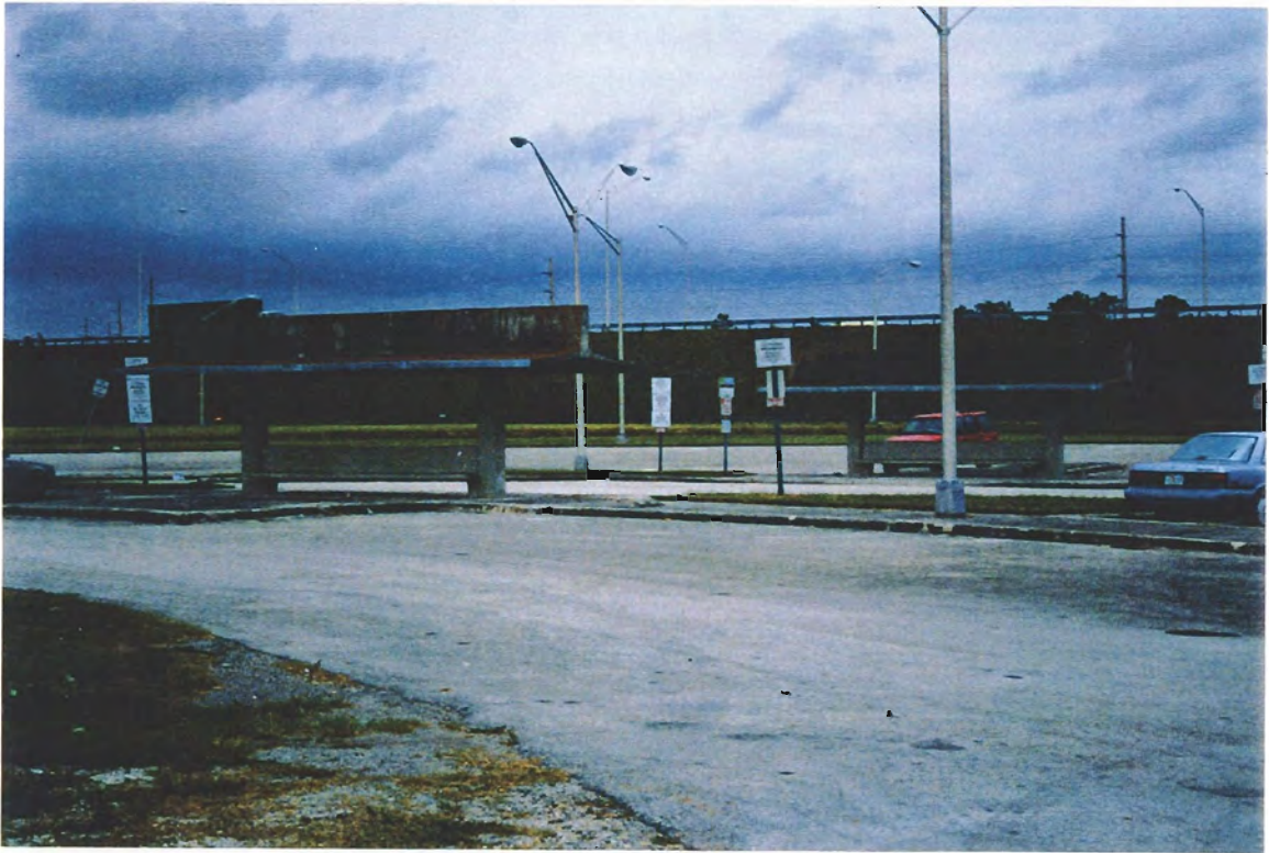
Northeast side view of existing bus stop, bay, and Park-n-Ride lot.
