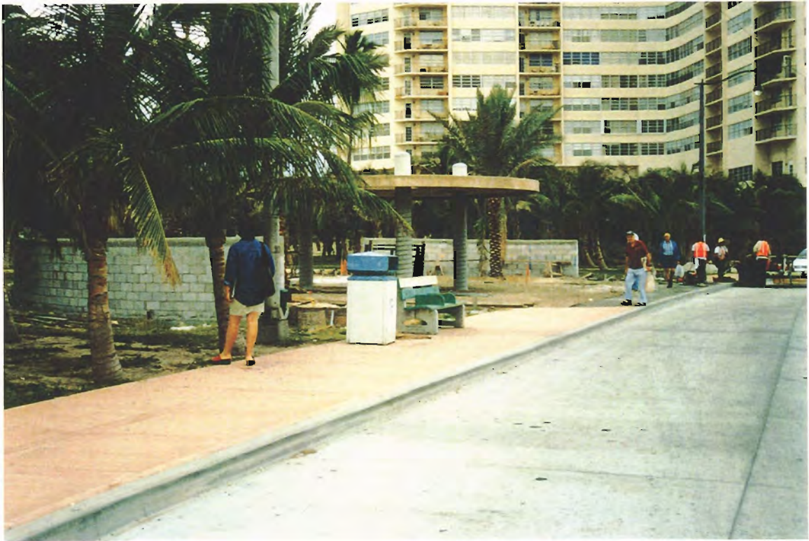
Intermodal facility under construction; view from the northwest.
