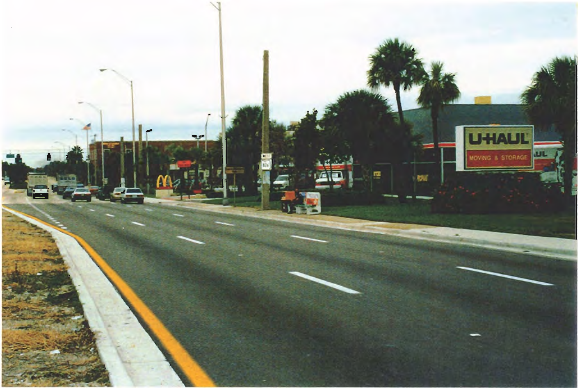
View of bus stop on 163rd Street (NW) and lane configuration.
