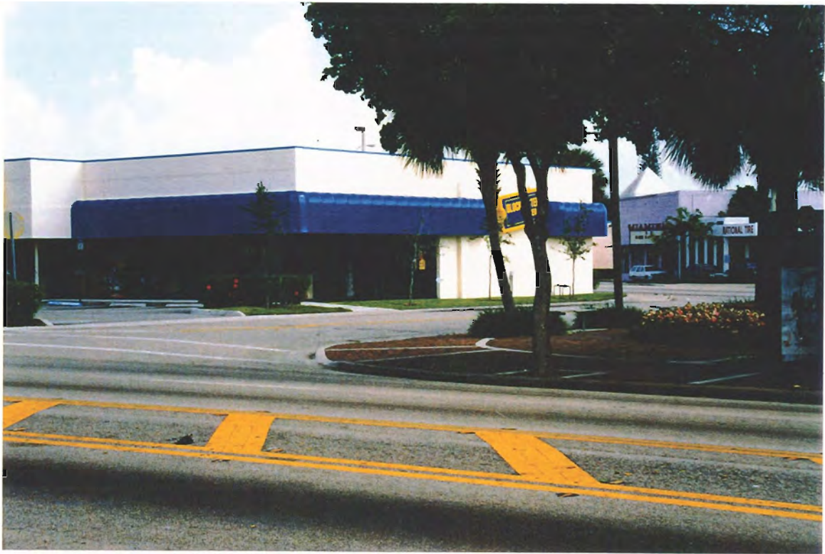
View of northern side of bus stop at Dixie Highway on 6th Avenue.
