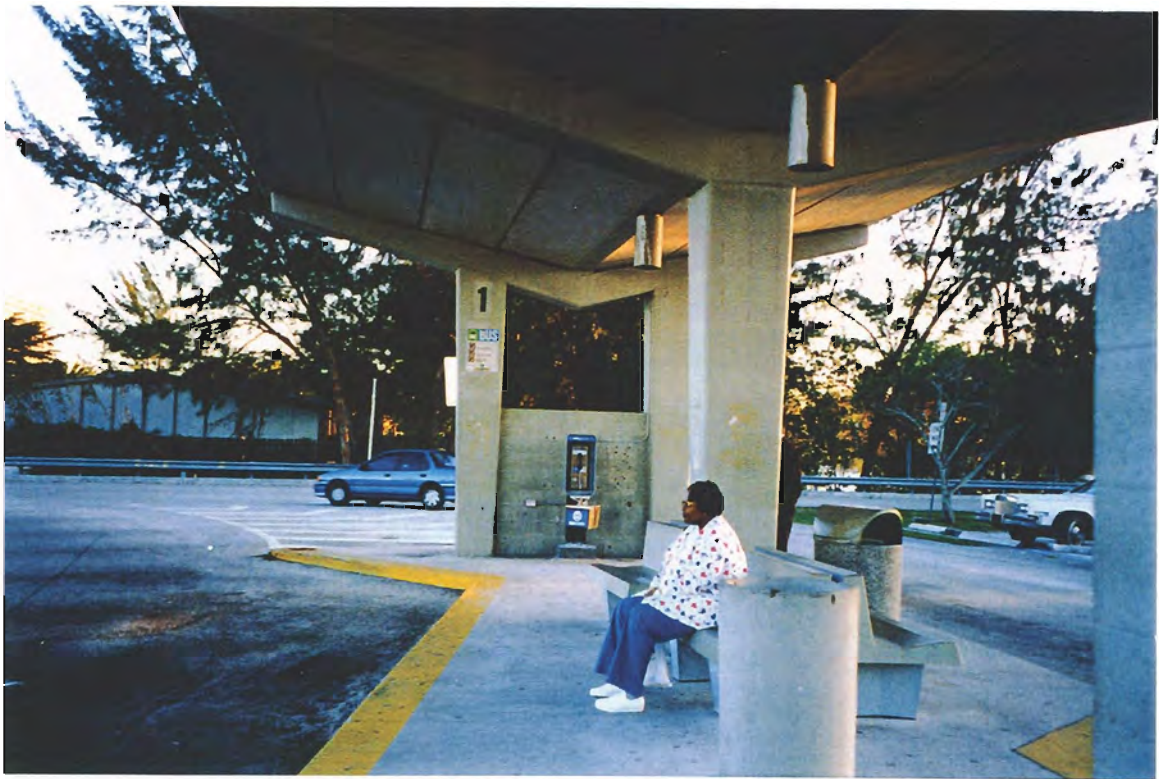
South view of bus terminal.
