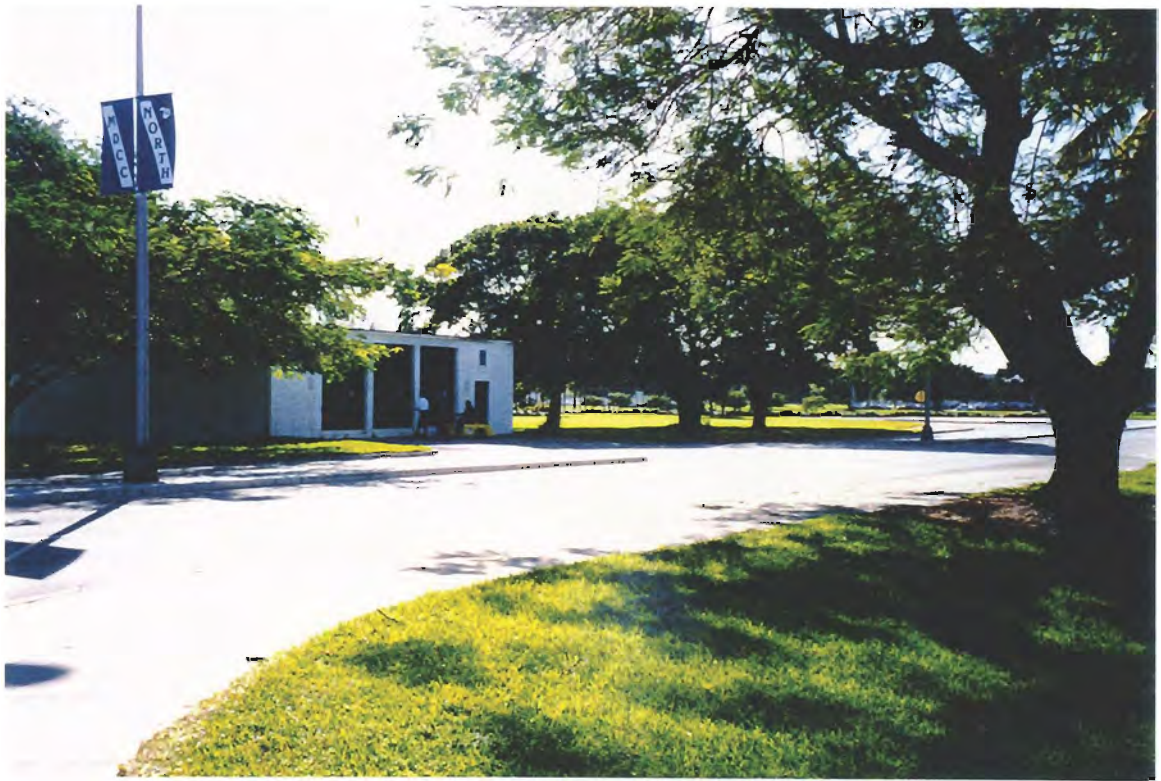
Southeast view of site location.
