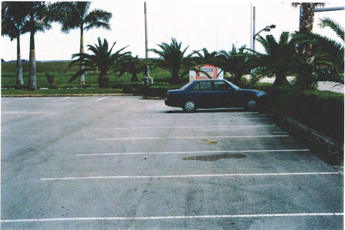
East side view of existing/future Park-n-Ride lot.
