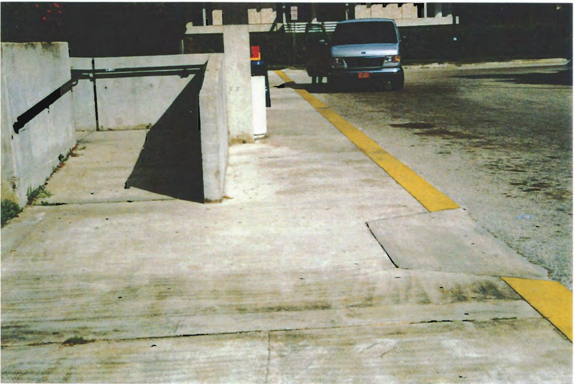
Curb cut ramp (west side of station).
