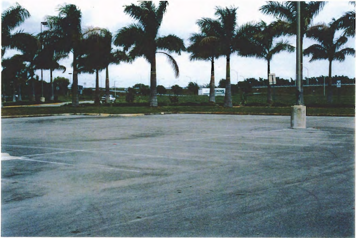
Northeast side view of existing Park-n-Ride lot.
