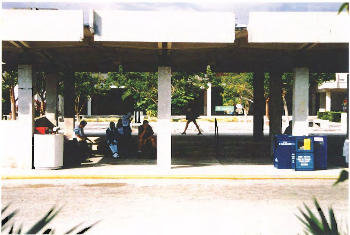
Bus stop (viewed from south).
