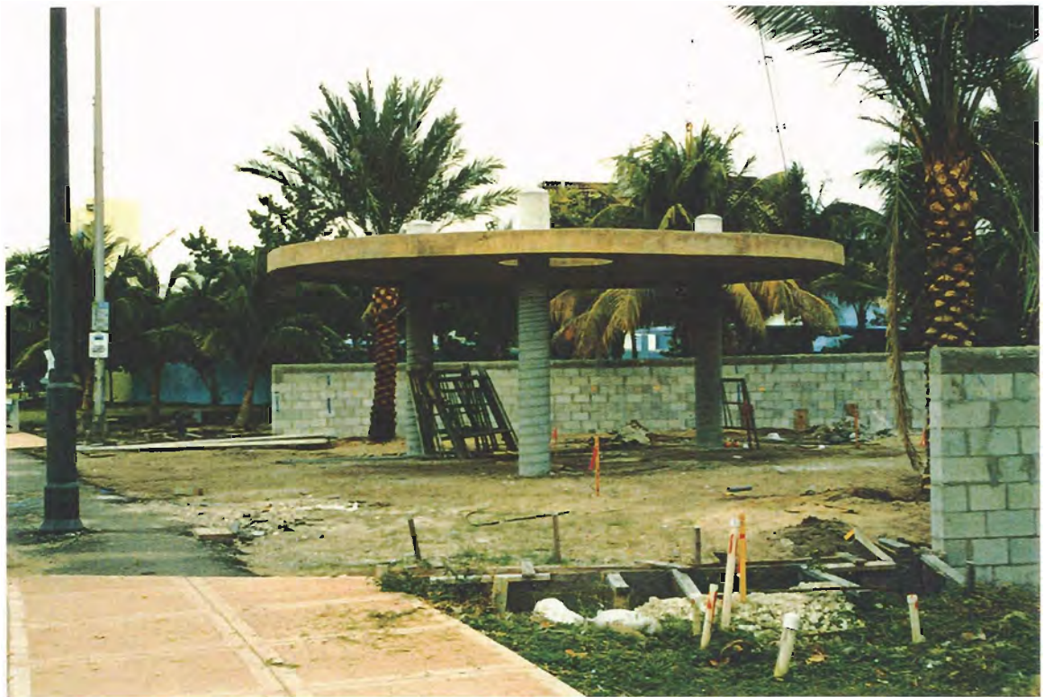
View of future terminal.
