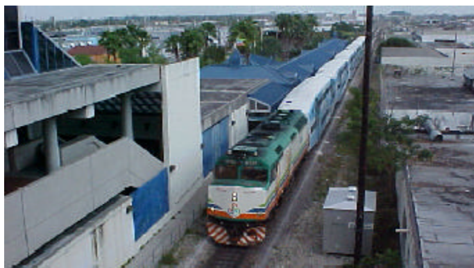
Existing Tri-Rail/Metrorail Transfer Station
