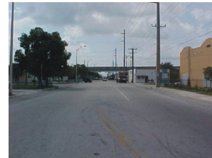
Existing NW 37th Ave. Looking South
