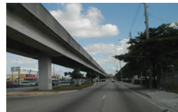
Eastbound NW 79th Street
