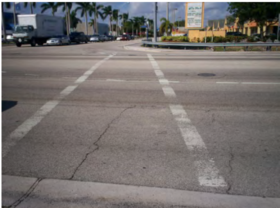
East leg: Lack of pedestrian features and ADA approved ramps.
