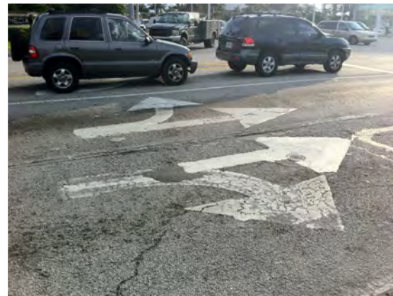
Faded pavement markings and deteriorated pavement conditions.
