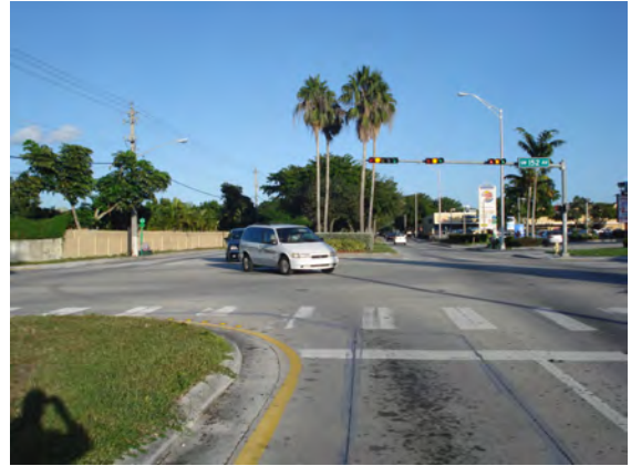
Eastbound/Westbound: Left-turn lanes are not aligned to reduce the offset.
