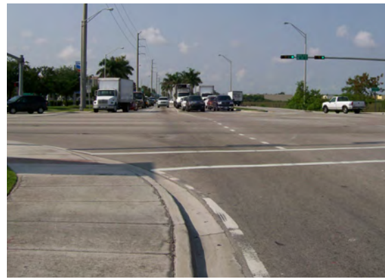
North/South: Road is not properly aligned with an offset to the left.
