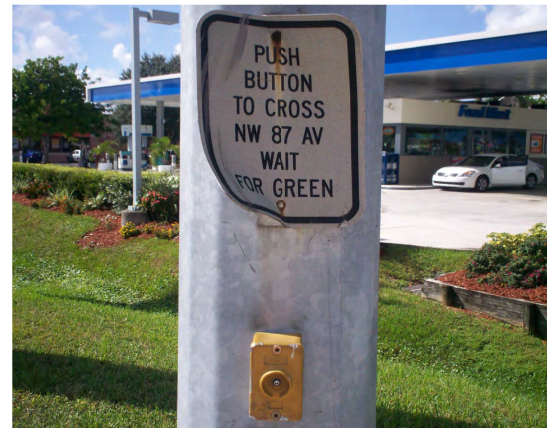
Damaged pedestrian features needs to be replaced.
