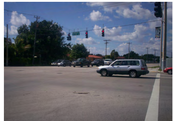
West & North legs: lack of pedestrian signal heads.
