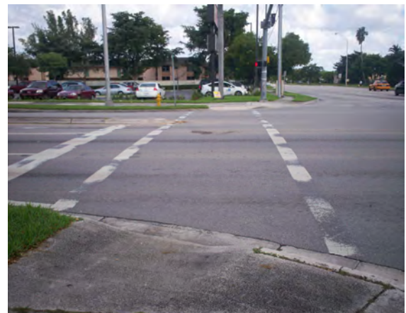
Faded pavement markings.
