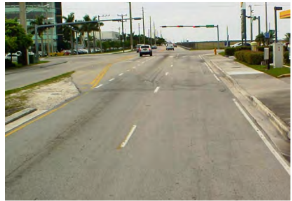
Westbound approach: Inadequate median length for left turn movement.
