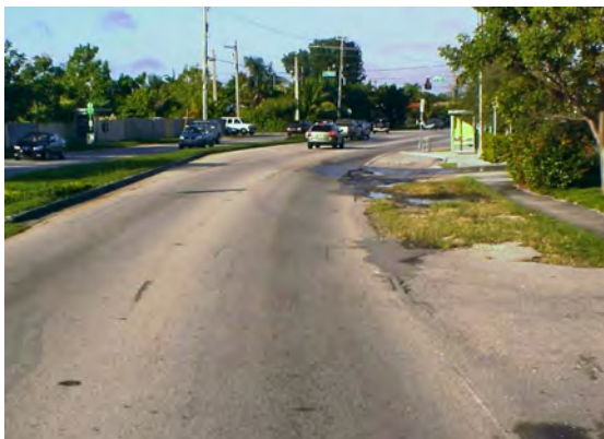
Westbound approach: Curve approaching a signal with no warning signs.
