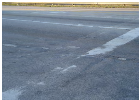
Faded pavement markings and deteriorated pavement conditions.
