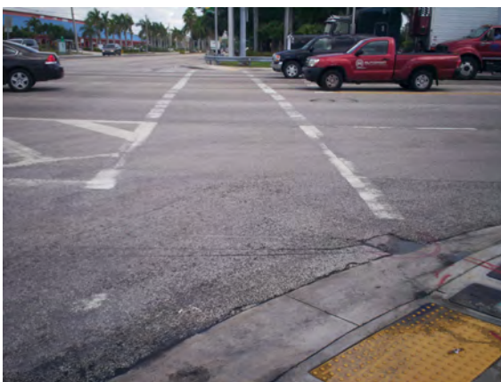
Faded pavement markings.
