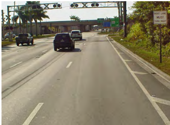
Southbound receiving lanes: No pavement markings to show the right-turn lane.
