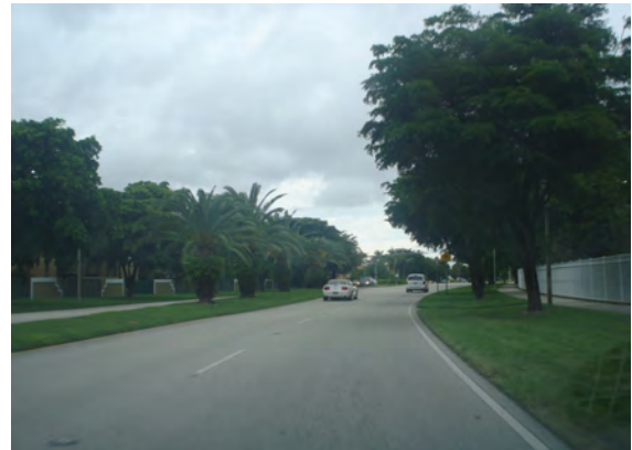
Northbound approach: No warning signs on the curve approaching a traffic signal.
