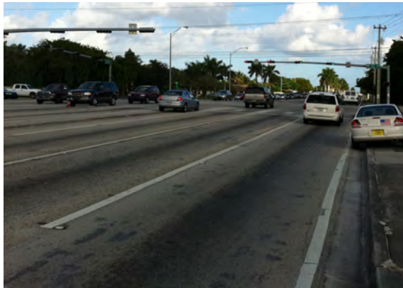
Eastbound approach: Deteriorated pavement conditions.
