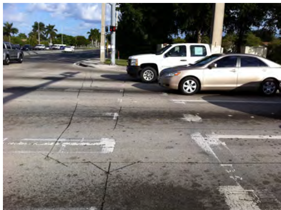
South leg: Faded pavement markings and crosswalks are too close to stop line.
