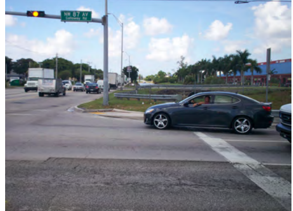
Southbound approach: Inadequate right-turn radius to handle heavy vehicles.
