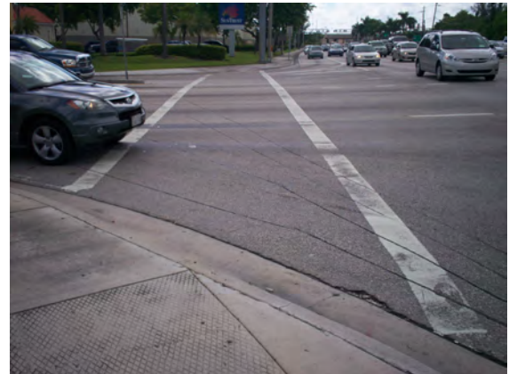
Faded pavement markings and no ADA approved pedestrian ramps.
