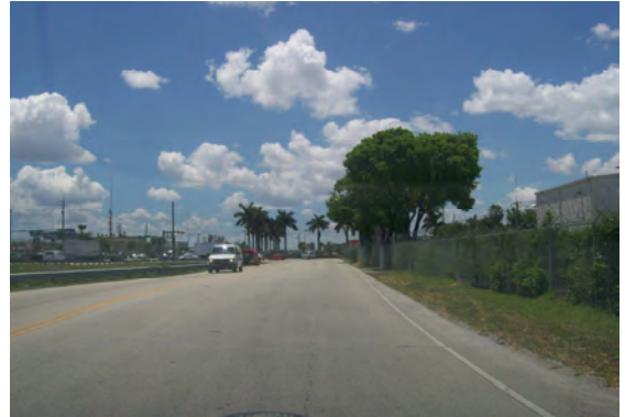
Southbound approach: Lack of warning signs to alert motorists of approaching a curve and a signal.
