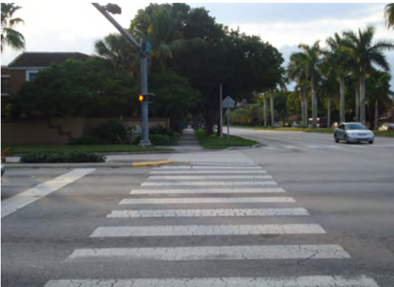
South Leg: Median nose obstructing the crosswalks.
