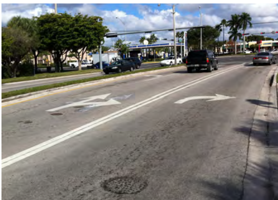
Eastbound approach: Substandard pavement markings.
