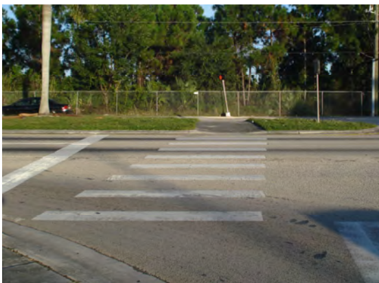
North leg: substandard pedestrian ramps and damaged signal post.
