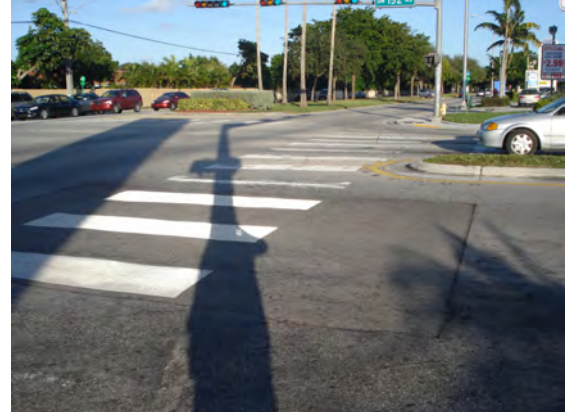
Faded pavement markings and uneven pavement patches.
