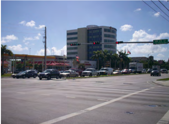
Northbound approach: Inadequate storage length to handle the heavy left-turn vehicles.
