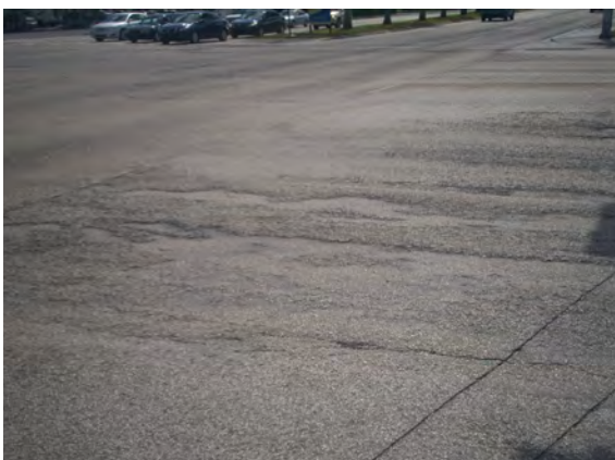
Deteriorated pavement conditions.
