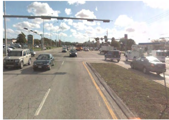
Northbound/Southbound: Left-turn lanes are not aligned to reduce the offset.
