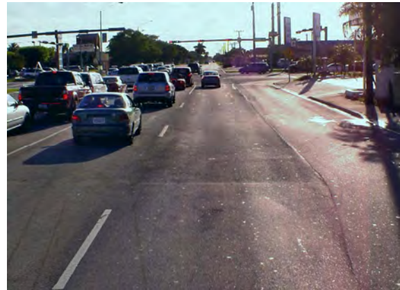
Eastbound approach: Right-turn lane with no pavement markings or signs.
