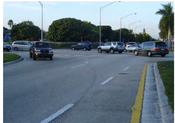
Eastbound right-turns: Inadequate channelization and tire marks.
