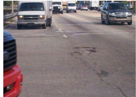
Faded pavement markings and deteriorated pavement conditions.
