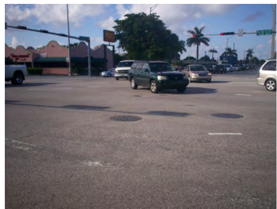
Faded pavement markings.
