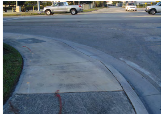
Southwest corner: Tire marks on the sidewalks indicating a tight turn radius.
