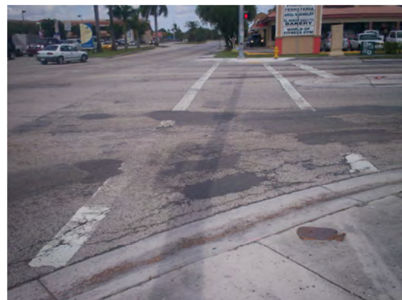
Faded pavement markings and deteriorated pavement conditions.
