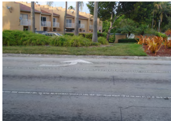
Faded pavement markings.
