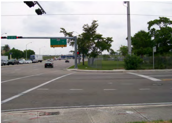
Northbound approach: Wide gap between the stop bar and the intersection.
