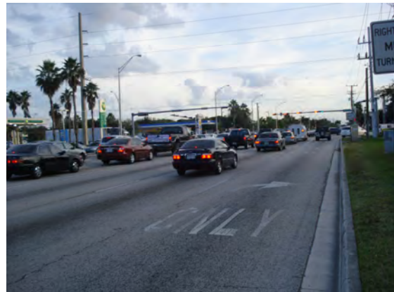
Southbound approach: Faded markings and deteriorated pavement conditions.
