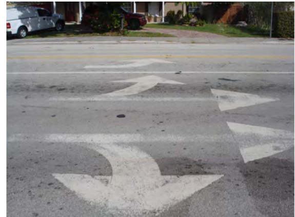
Faded pavement markings and deteriorated pavement conditions.
