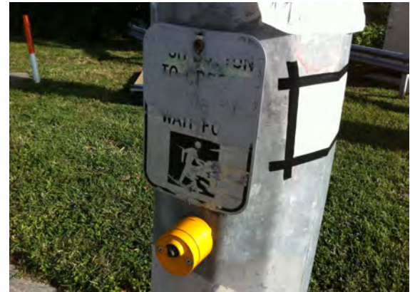
Southeast corner: Pedestrian sign needs to be replaced.
