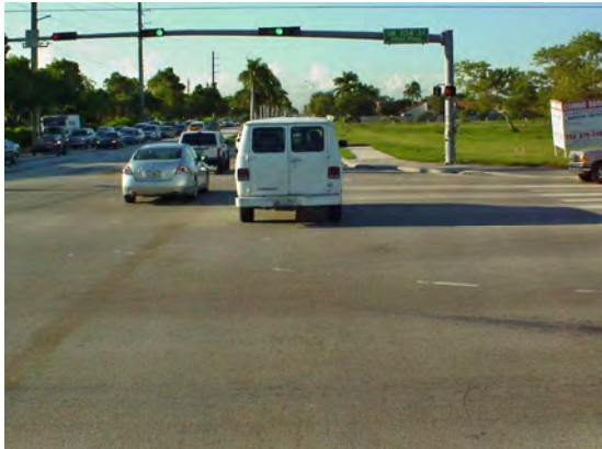
Faded/No double left-turn guidelines at the intersection.
