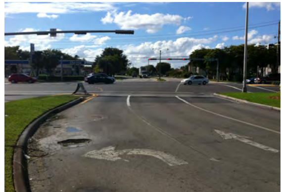
Westbound approach: Faded pavement markings and deteriorated pavement conditions.
