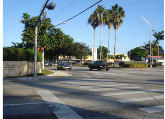
Northeast corner: Sight distance issue and tight turn radius.
