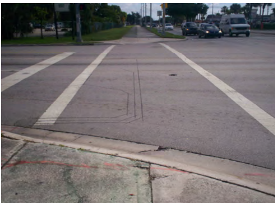
North leg: Lack of ADA approved pedestrian ramps.
