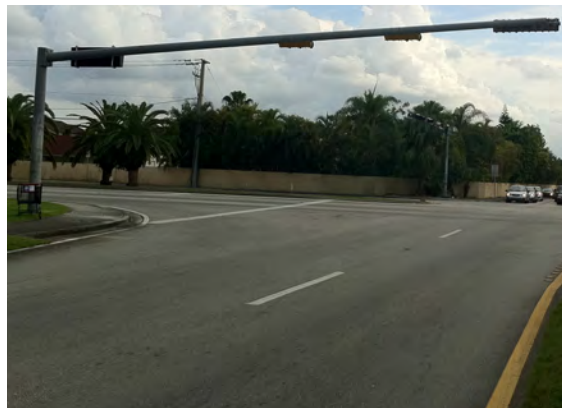
North leg: Lack of ADA approves pedestrian ramps and pedestrian features.
