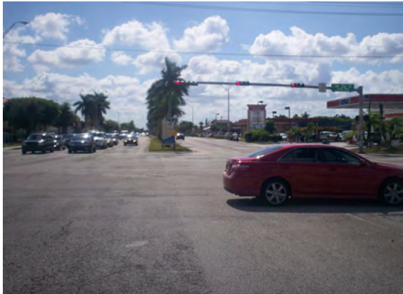
Northbound/Southbound: Left-turn lanes are not aligned to reduce the offset.
