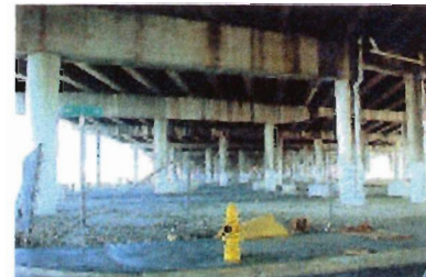
Horrific conditions beneath I-395
