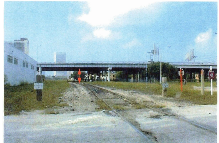
A clearance of 23.5 feet is required between the tracks and I-395
