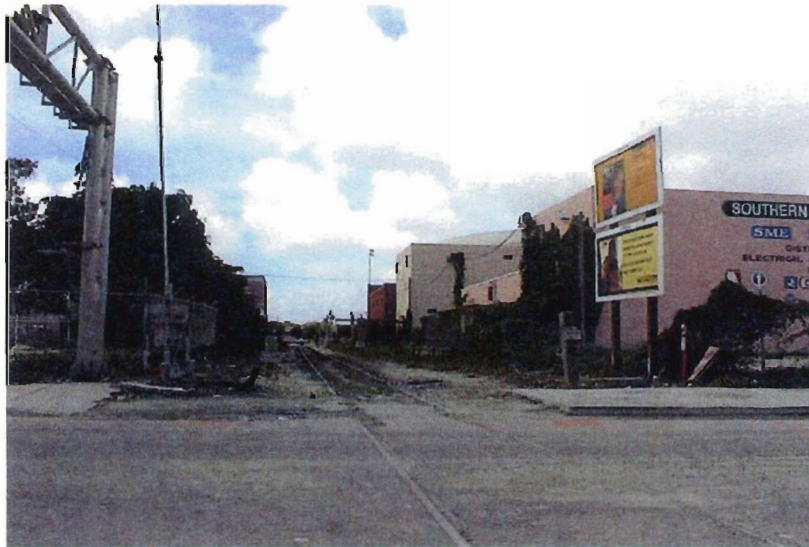
View of the FEC tracks towards Wynwood
