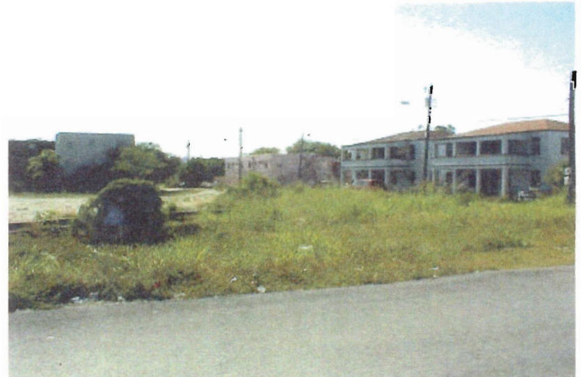
Empty lots and dilapidated housing in Overtown
