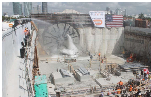
Figure 3-9 Breakthrough of First of Two PortMiami Tunnel Bores
